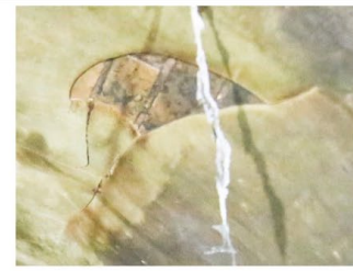
Figure 2: Feature - Closeup of debonded epoxy coating
