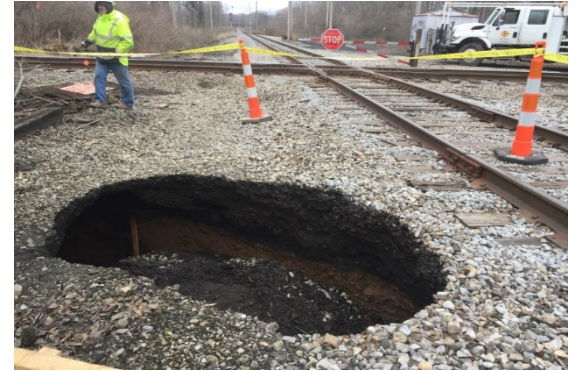
Sinkholes under railroad
