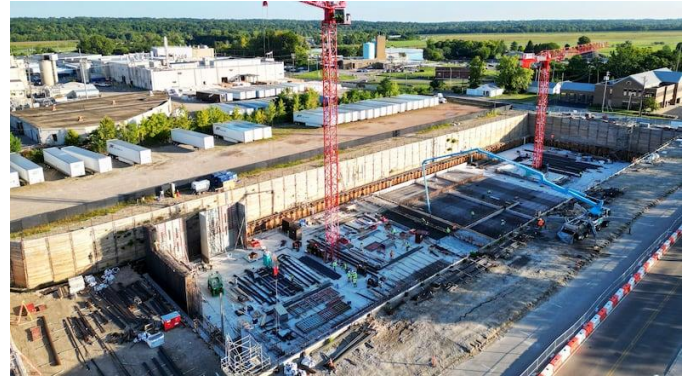
Construction of Underground EQ Storage Tank
