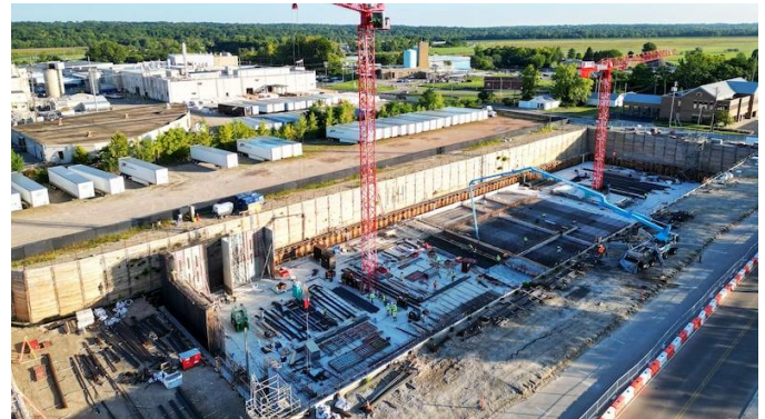
Construction of Underground EQ Storage Tank
