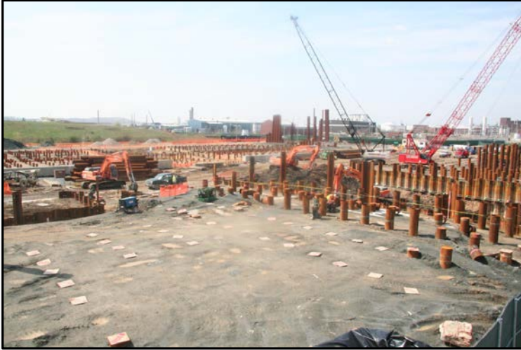
Denite filter pile driving – April 2011
