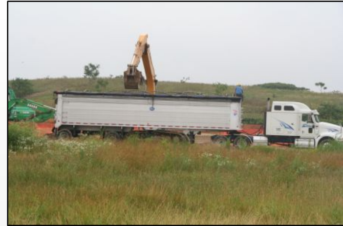
100% excavated soil removal
