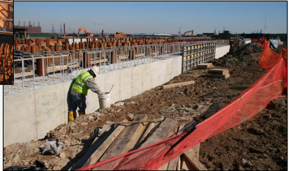
40,000+ cy of concrete to be placed including the grade beams for the BAF structure
