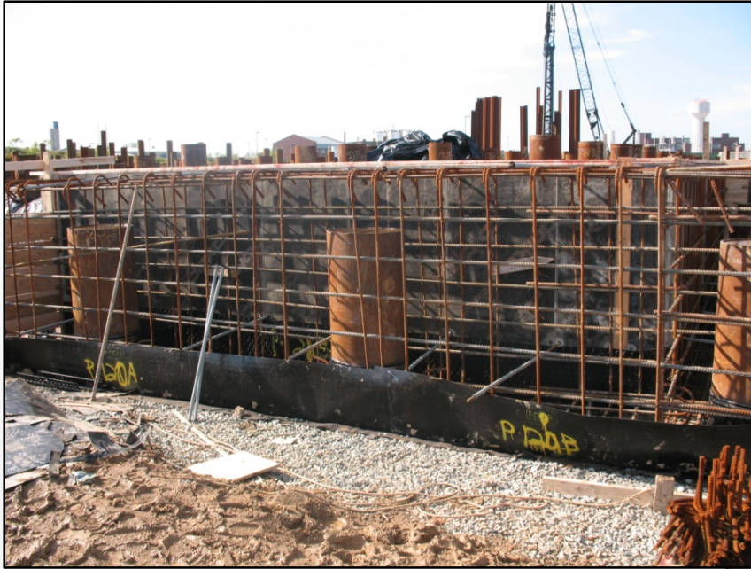
24 in steel pipe pile to be embedded in the concrete foundation for all structures
