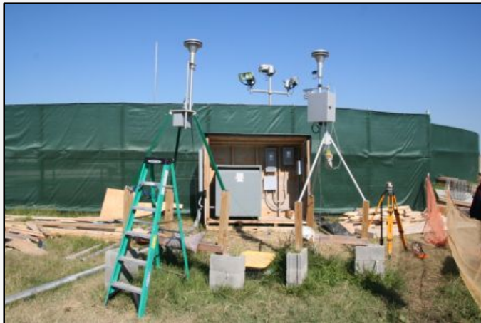
24 hr. air and dust monitoring
