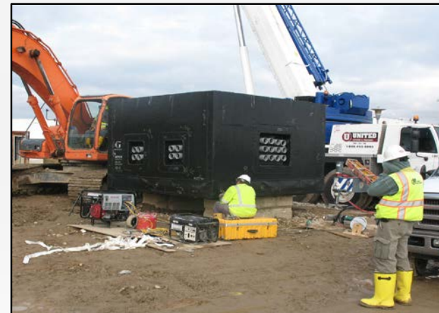
HDPE liner on all structures below groundwater
