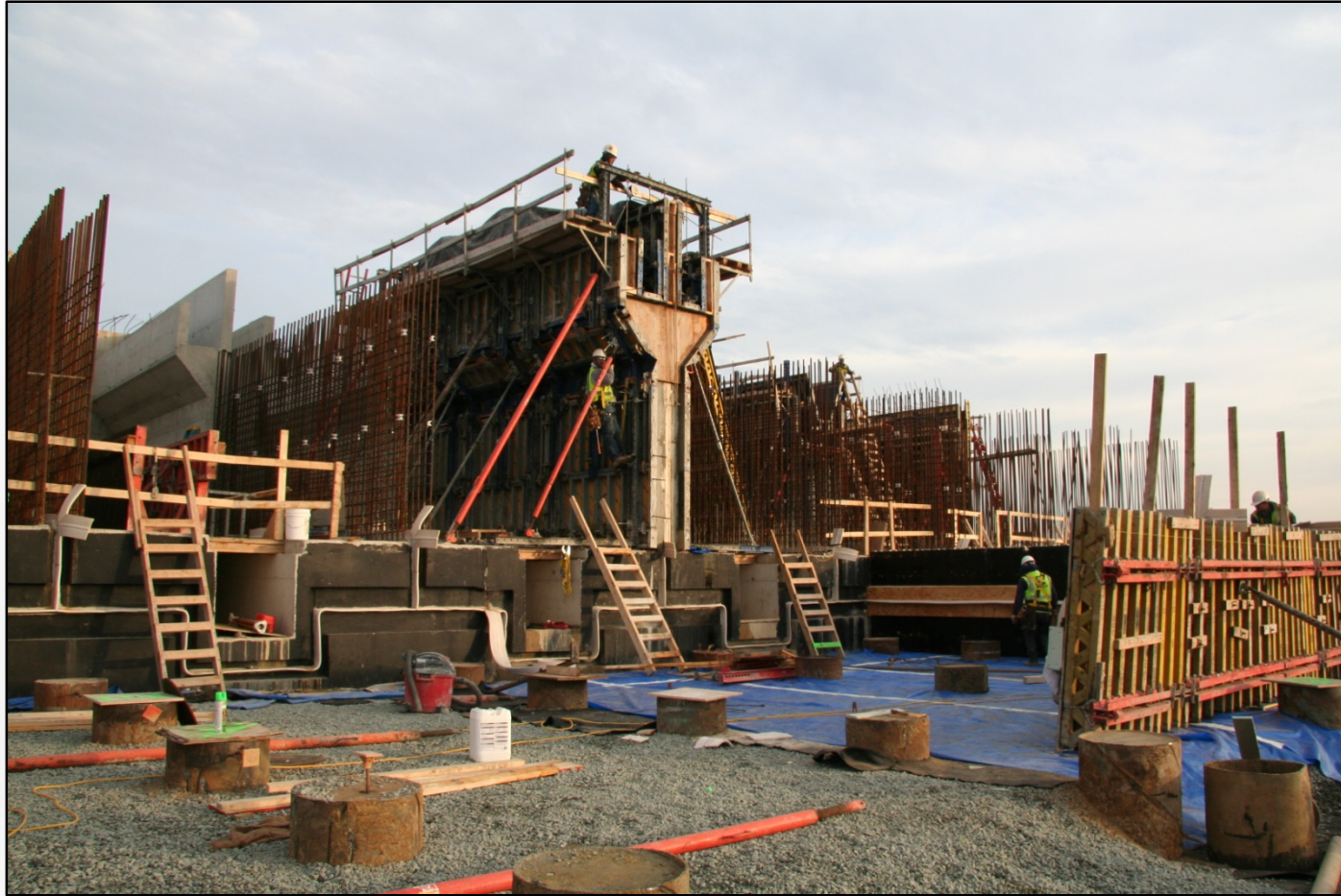
DNF gallery detailing the extensive formwork necessary to construct
