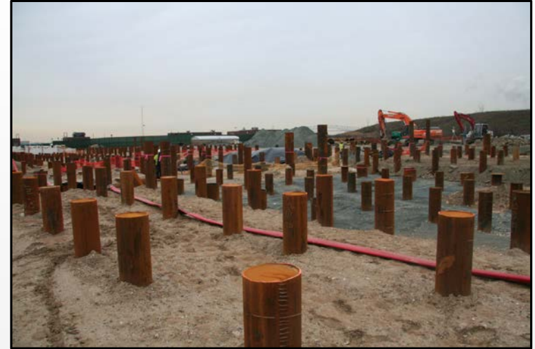
More than 1,100 piles later, BAF pile driving
