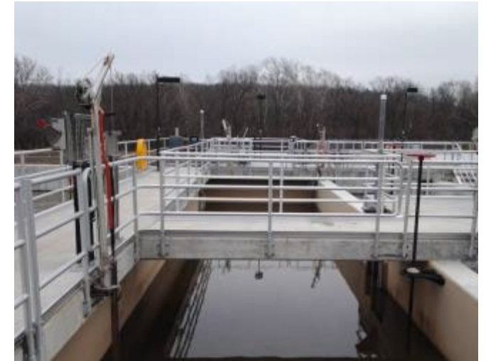
Off-line Mixed Liquor Fermenter with 5-stage Bardenpho 5.3-mgd Cedar Creek WWTP (Olathe, Kansas)
