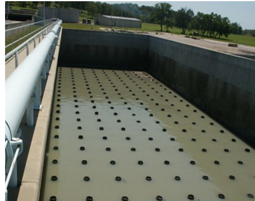
Offline Biomass Storage Rogers, Arkansas 5-stage Bardenpho Oxidation Ditch
