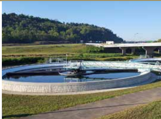
Wastewater Treatment Plant | Athens, OH
