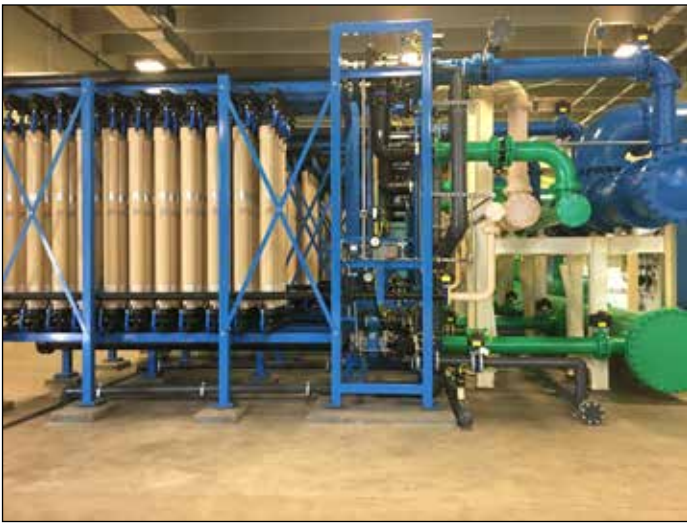
Equipment such as membranes require multiple header pipes to be positioned nearby and can result in the need for custom pipe support structures.
