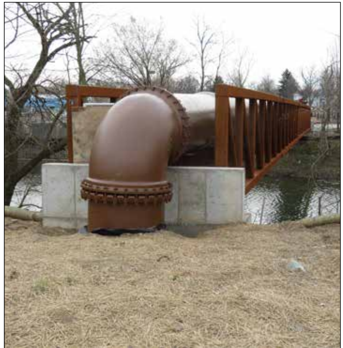
Completed overland river crossing of a 42" force main.
