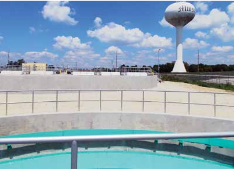
Ohio's Minster Wastewater Treatment Plant Upgrade and Expansion was constructed in 2012, with solids handling improvements in 2015. Current capacity is 1.27 MGD, with a peak flow of 4.82 MGD.
