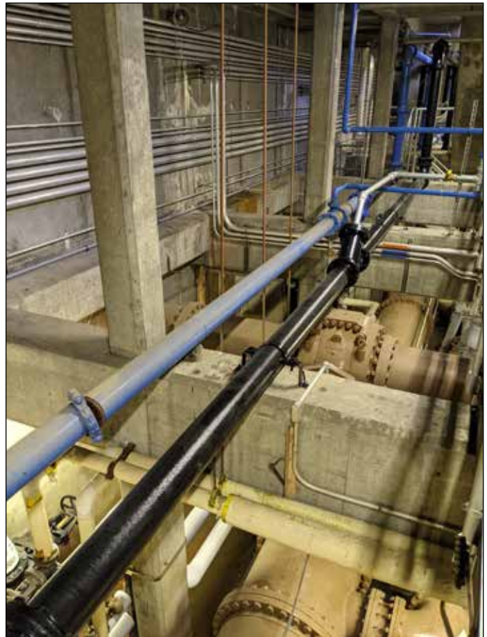
Not giving piping design the attention it deserves can lead to early failure of pipe joints.
