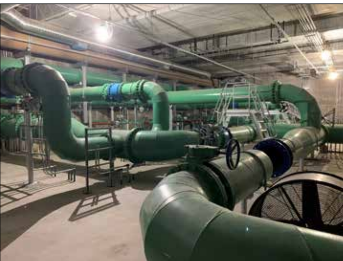
Creative piping design can lead to flexibility in raw water source blending ahead of pretreatment.
