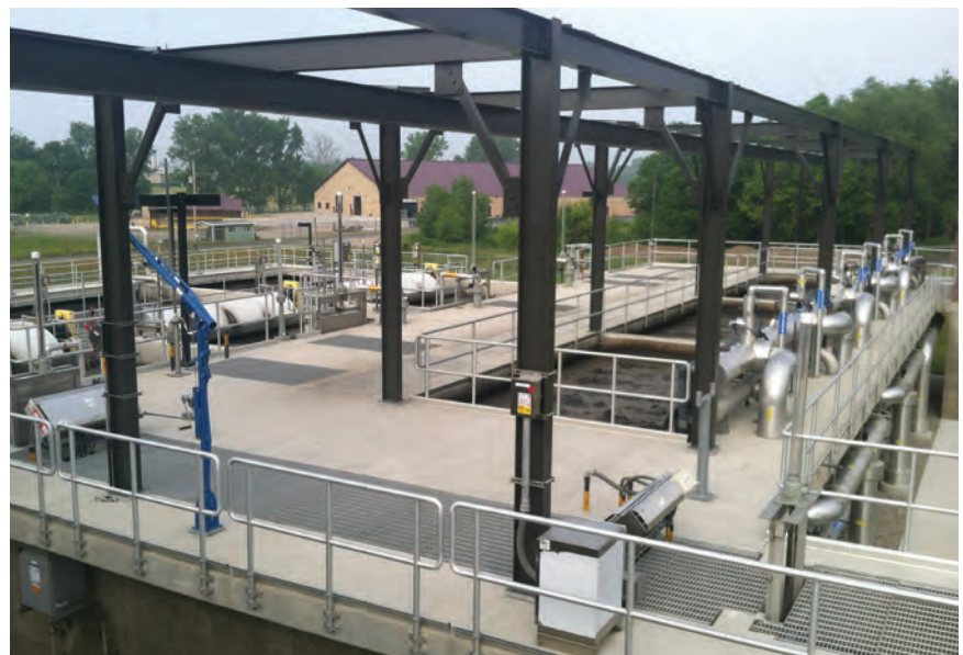
Secondary treatment facility
