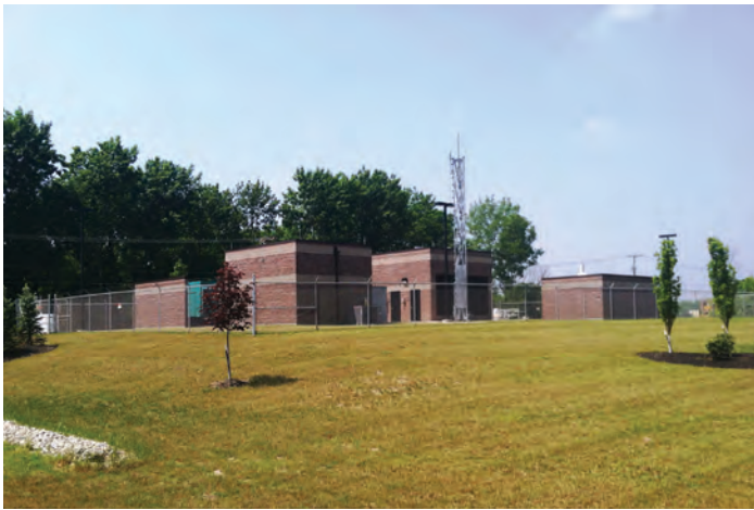
Upper Hocking Pump Station
