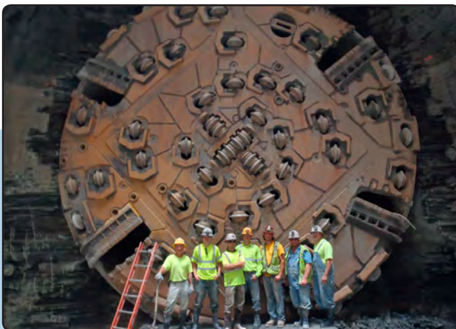
NORTHEAST OHIO REGIONAL SEWER DISTRICT EUCLID CREEK TUNNEL
