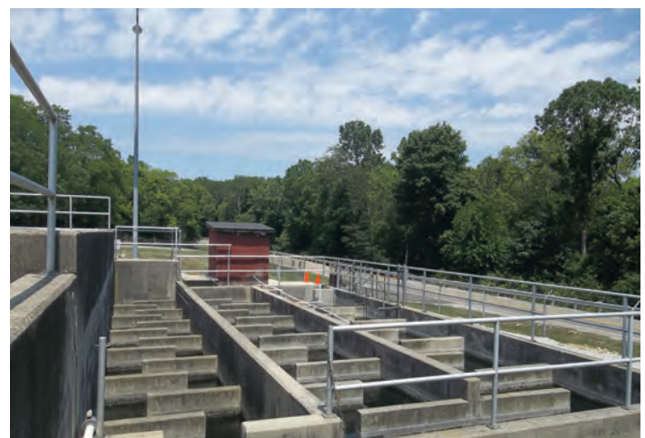
Chlorine contact tank
