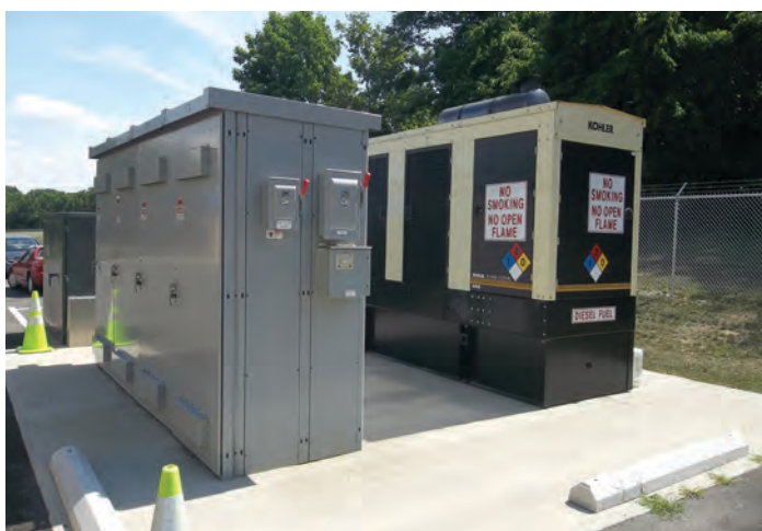
Transfer switch and generator
