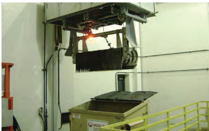
Brackett Green Sewage Bosker screen raking assembly at the St Louis WWTP installed as part of the Lower Meramec River System Improvements project. (St. Louis WWTP)
