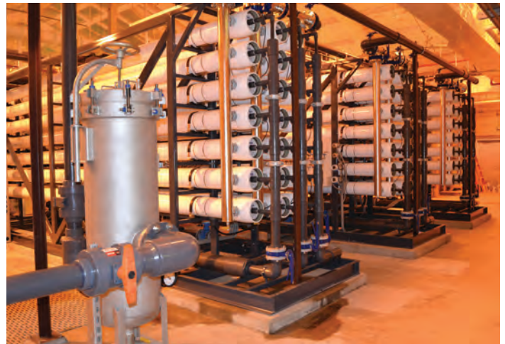
This is the newly installed reverse osmosis system at the Pickerington Water Plant.
