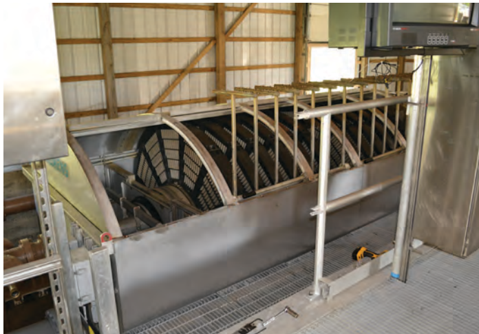
Photo of disc filters which were installed as part of the 2009 expansion. They replaced sand filters as the means of tertiary treatment.
