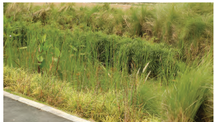
Rainwater passes through the rain garden, and the filtered water then flows into the stormwater drain.
