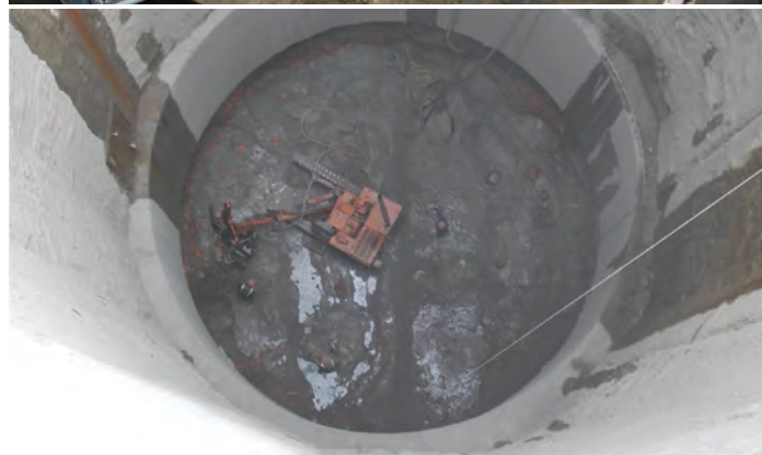
(Top to bottom) (1) CSM (cutter-soil mix) wall construction provides a water-tight excavation protection system in the soft ground portion of Shaft 1, for the foundation slab of the upper ring channels on the diversion structure. (2) A clamshell bucket used for the excavation of the CSM wall and slurry wall. (3) Excavating the soft ground in Shaft 2 within the slurry wall excavation support system. (4) Preparing for blasting in Shaft 2 to continue excavating in the rock. (DLZ Ohio, Inc.)
