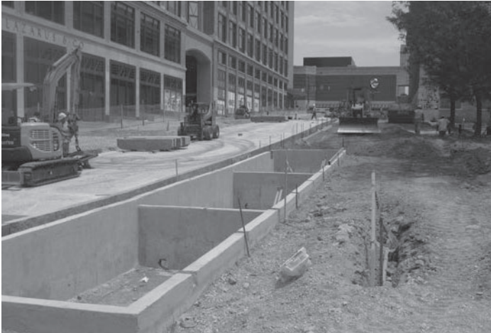
Constructing bioretention basin
