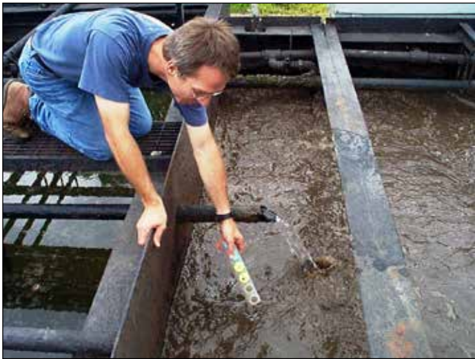
Figure 5: Sampling the Effluent End of the Aeration Tank
