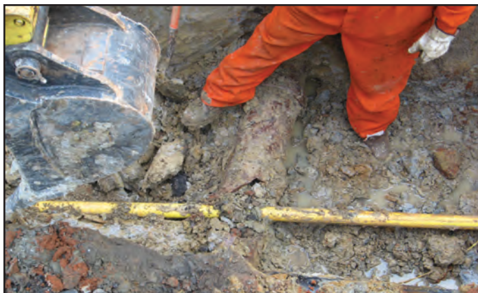
Figure 13: Gas line through the sanitary sewer. Most likely cause of the observed I/I. Other minor sources were documented
