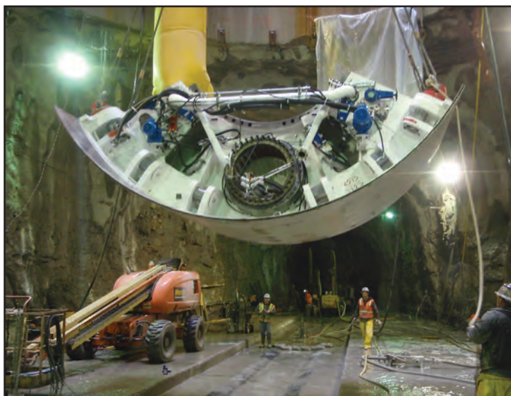
Lower 1/3 rd section of front shield of TBM. Columbus, Ohio OARS Tunnel project
