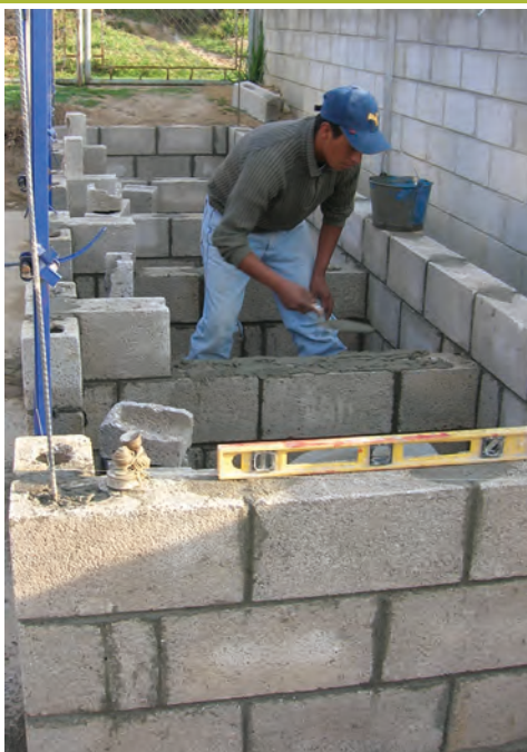
A local mason builds the walls of a latrine in Quiché, Guatemala. (John Niewoehner, WFP Photo)
