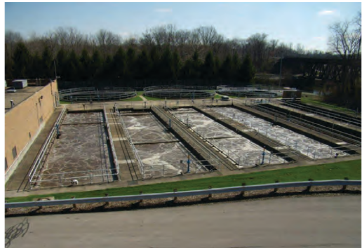
Aeration tanks and secondary clarifiers
