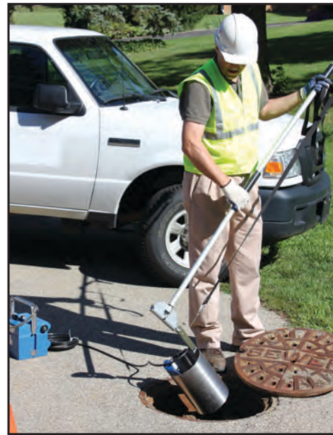
Figure 9: The micromonitor can be installed from the surface without CSE.
