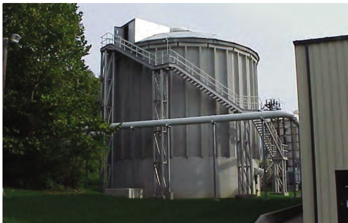
Trickling Filters
