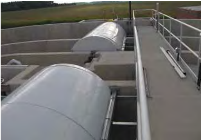
View from above Orbal, showing aeration rotor covers.
