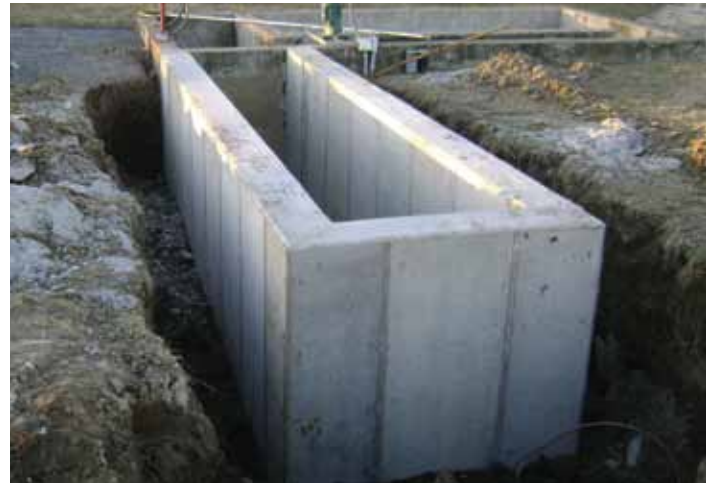
Construction of the UV disinfection channel with the existing chlorine contact tank in the background.
