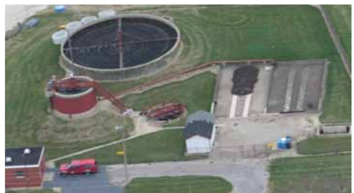
Aerial photograph of original wastewater treatment plant, showing pump station, Spiragester, trickling filter, clarifier, chlorine contact tank and sludge drying beds.
