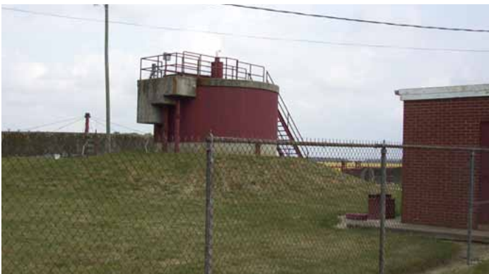
Original wastewater treatment plant, showing pump station in foreground and Spiragester and trickling filter in background.
