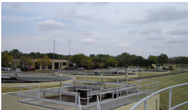
Splitter box and final clarifiers
