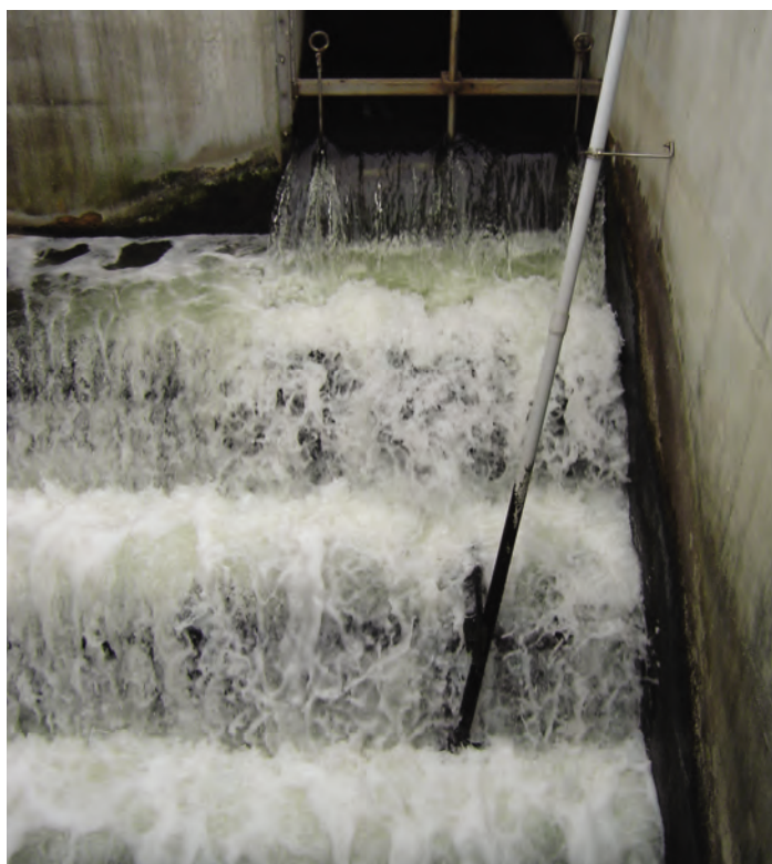
Cascade aeration of the final effluent
