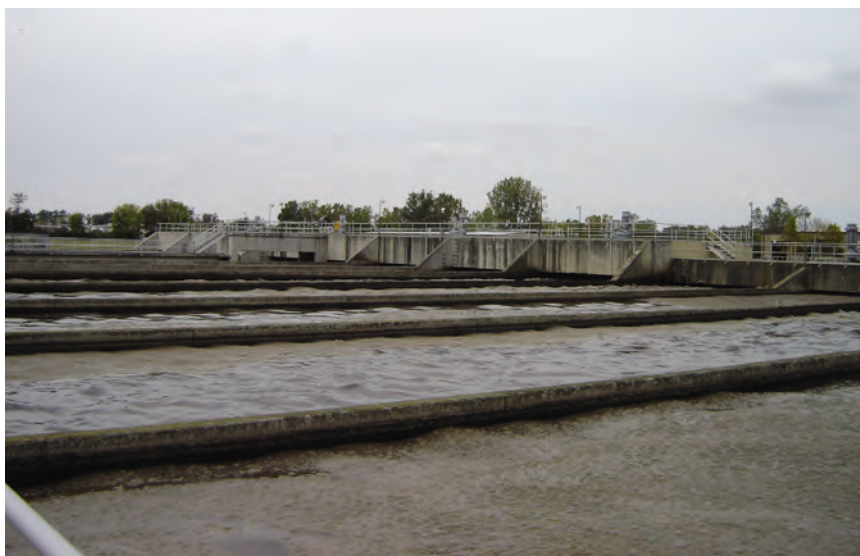
Oxidation ditches
