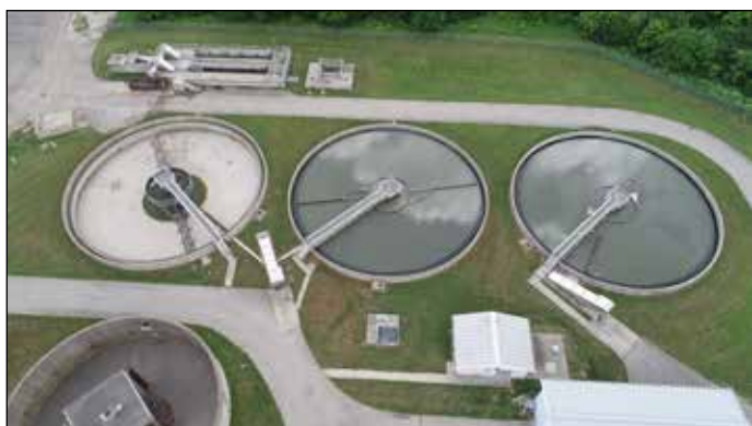
Aerated Grit Tanks and Primary Clarifiers
