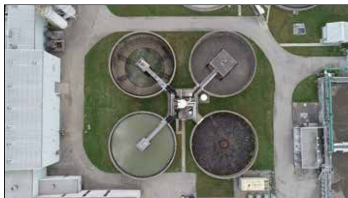
Sludge Thickeners
