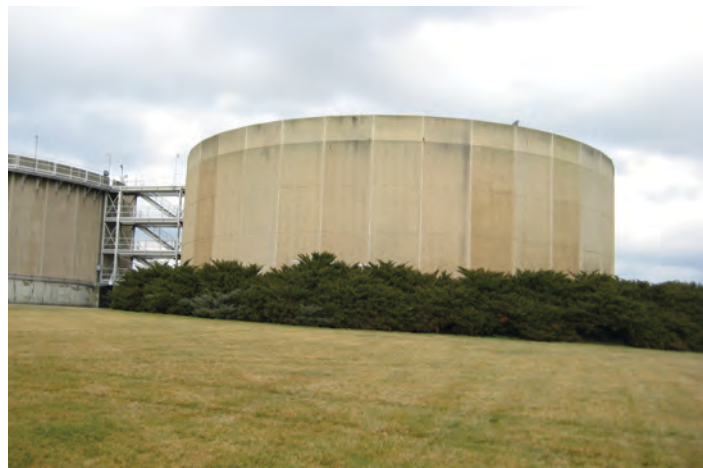
Trickling filter in operation
