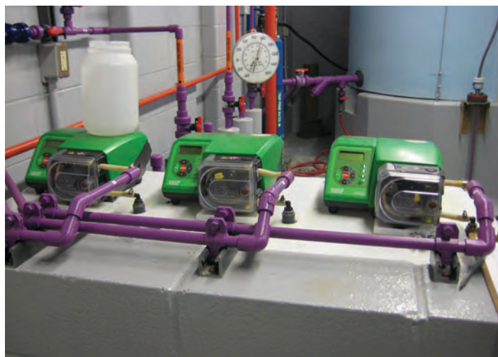
Ferric chloride feed pumps
