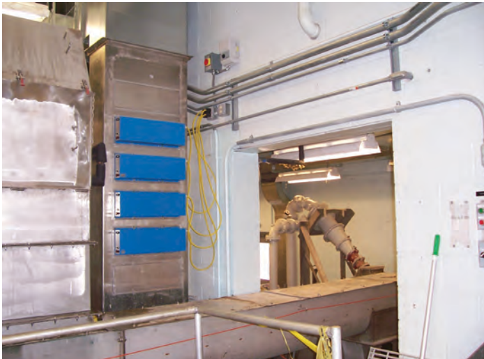
Figure 2: Port Clinton WWTF Headworks Air Ionization Unit (AIU) Plenum
