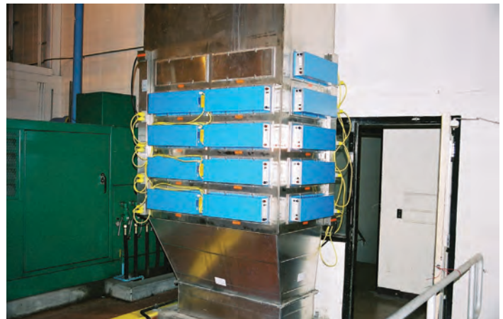
Figure 4: Denver Metro Air Ionization Unit (AIU) Plenum
