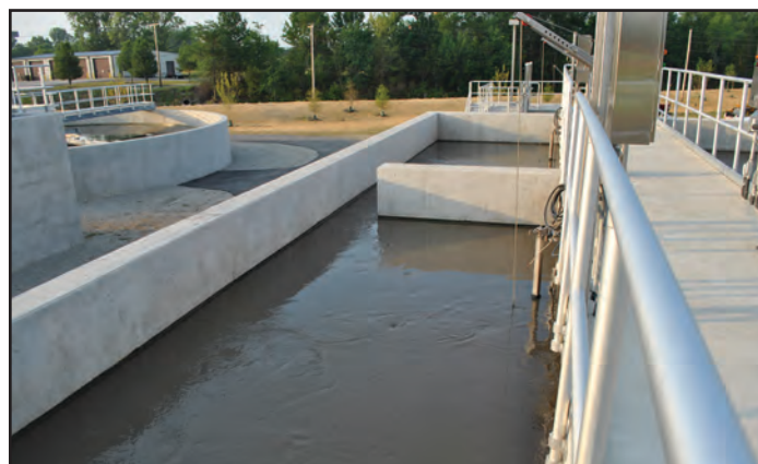
Figure 2: Anaerobic Zones for EBPR
