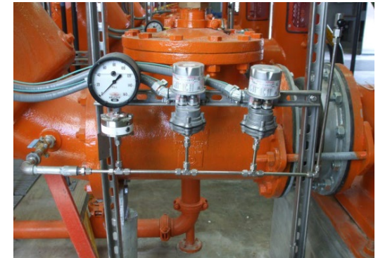
Non-Potable Pressure Gauge
