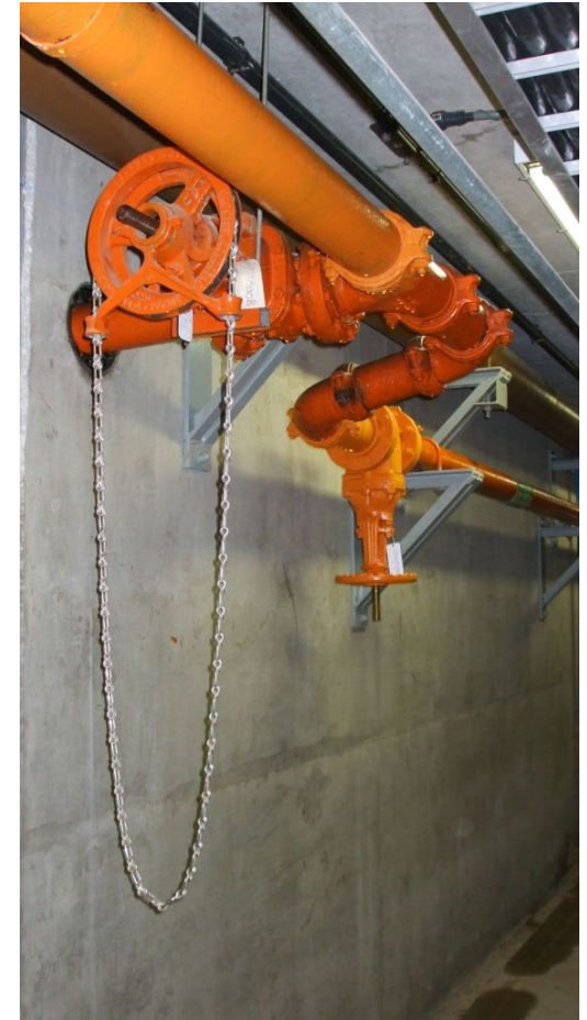
Non-Potable Water Header
