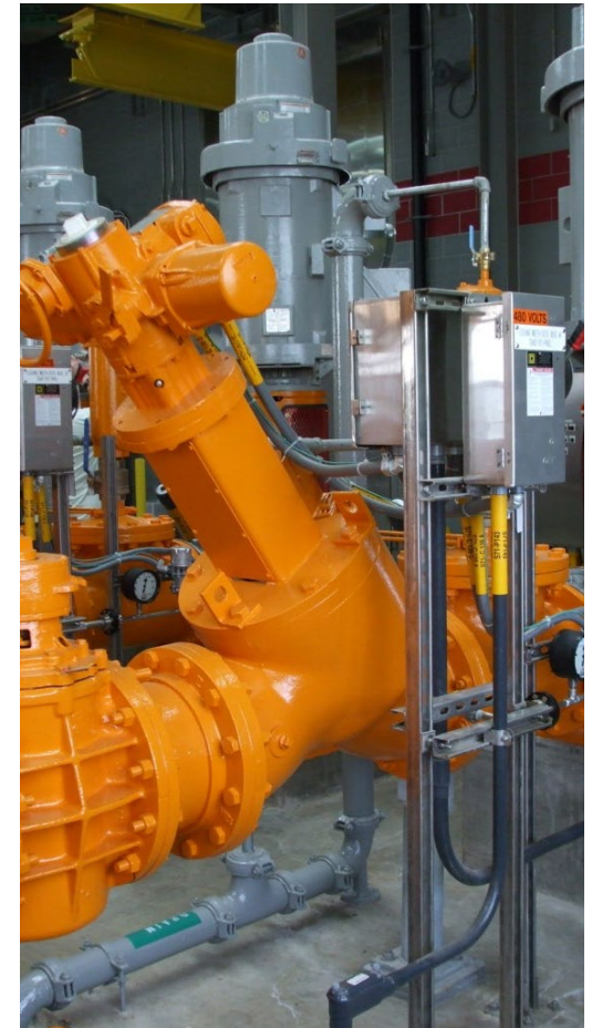
NPW Pump Check Valve
