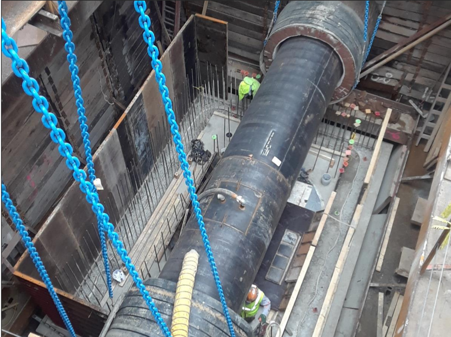
Jefferson / Superior Drop Shaft Construction
