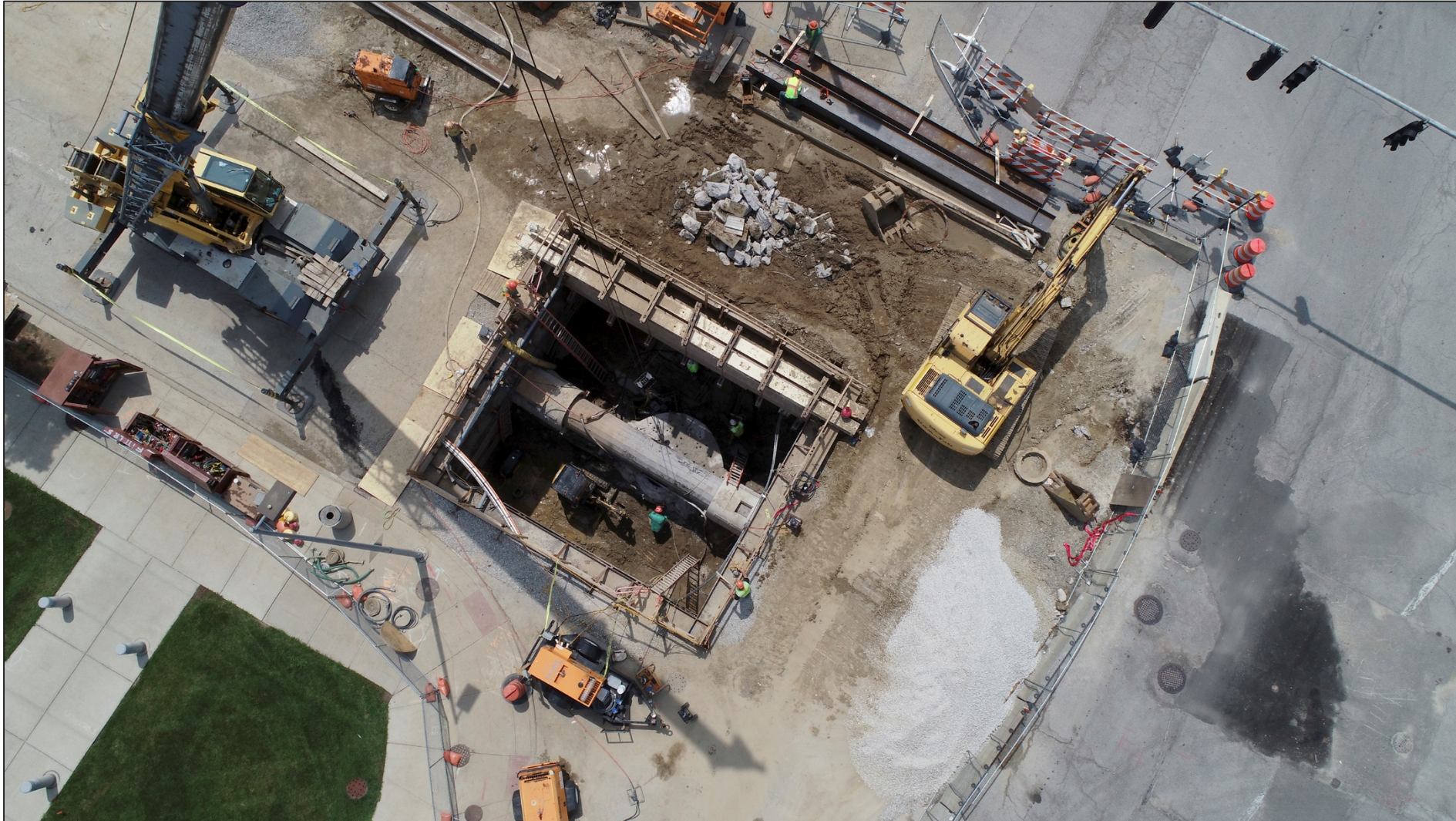
Jackson / Superior Drop Shaft Construction Photo Taken by David Patch, Photographer for The Toledo Blade
