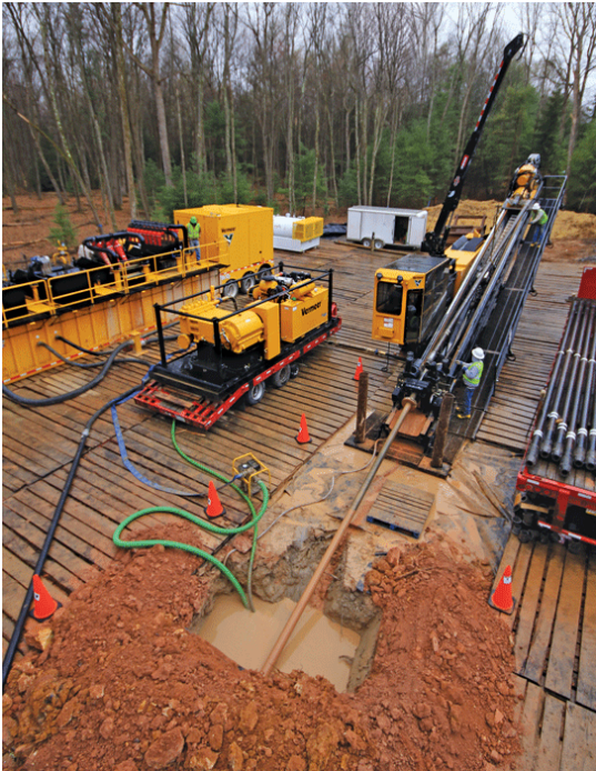
Horizontal Directional Drilling
