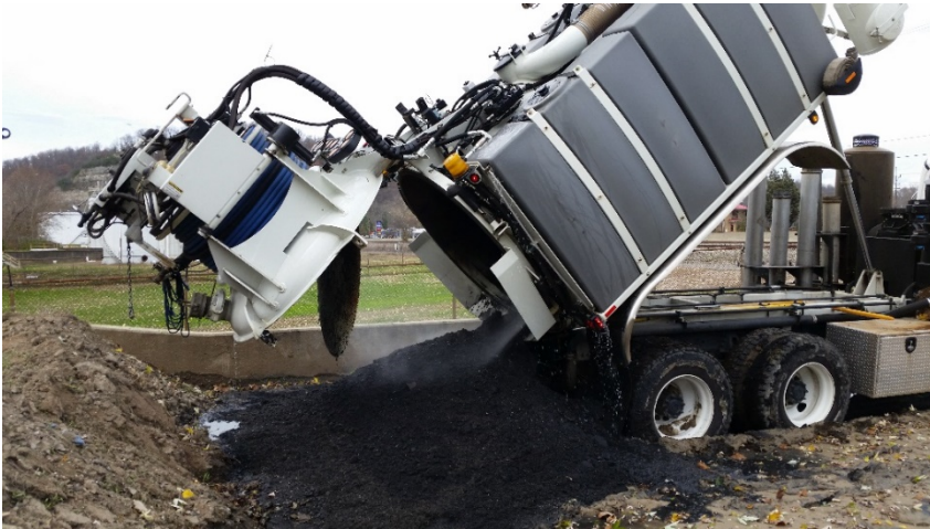
Courtesy of: Strand Associates, Inc. ®
