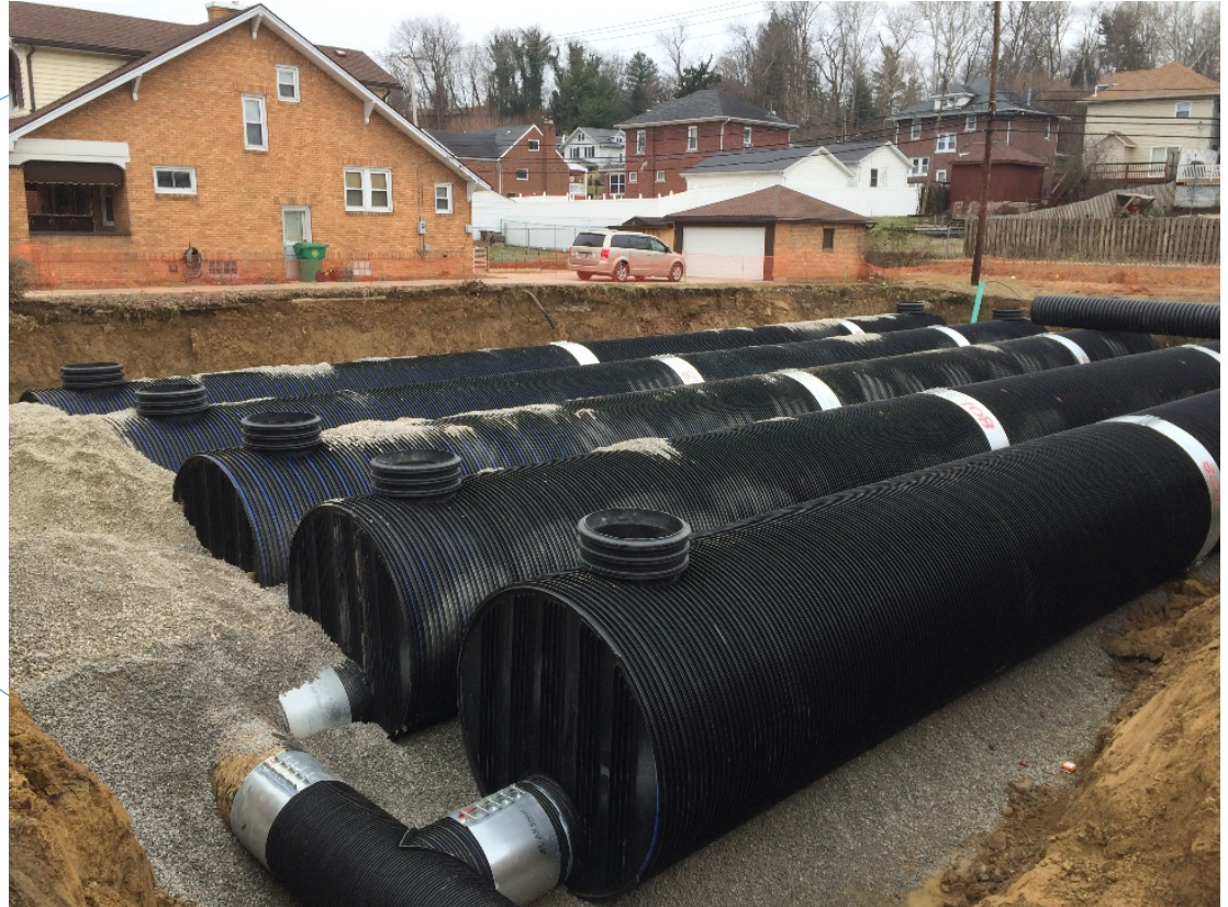
Courtesy of: Strand Associates, Inc. ®
