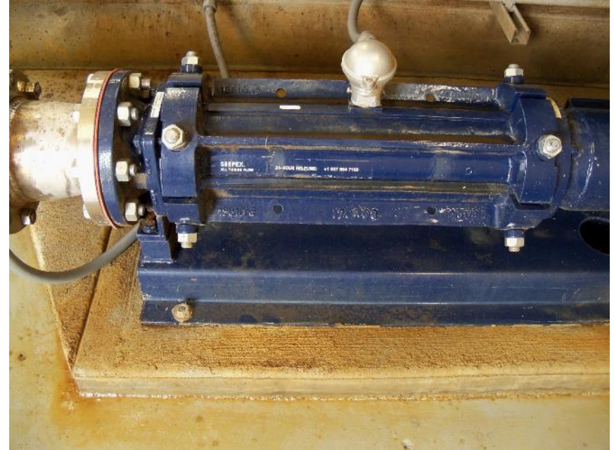
Thickened Sludge Pumps Seepex Progressive Cavity
