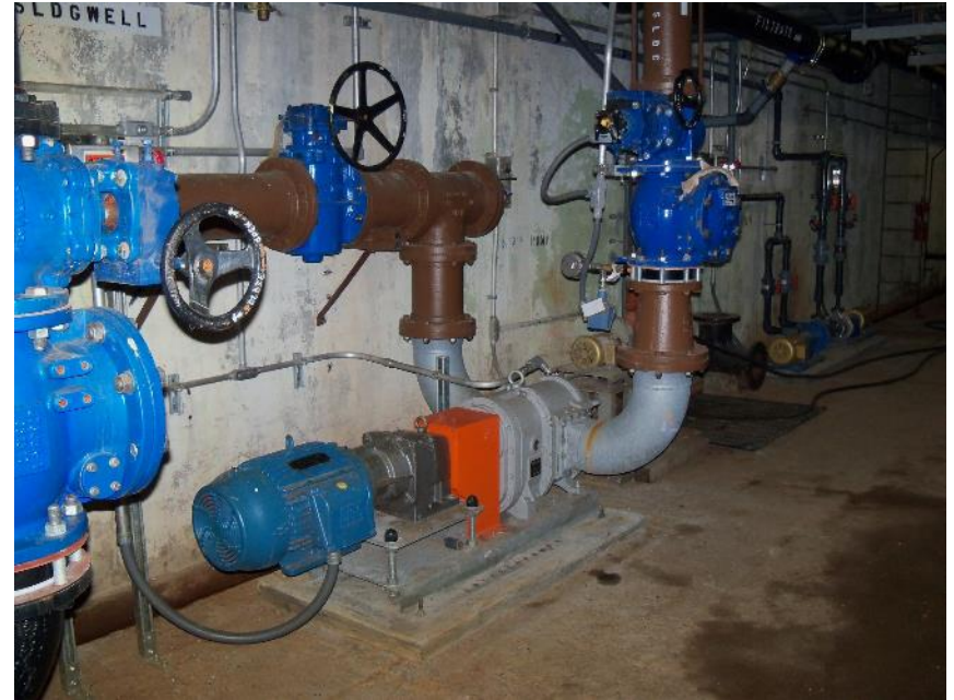
GBT Feed Pumps Boerger Rotary Lobe
