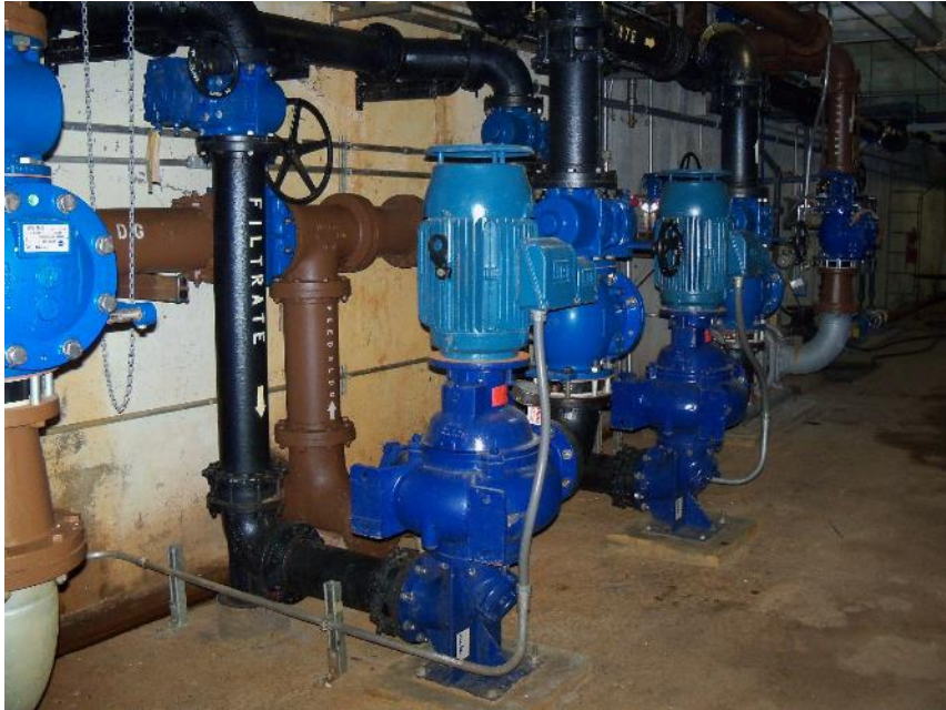
Filtrate Pumps KSB Dry Pit Centrifugal
