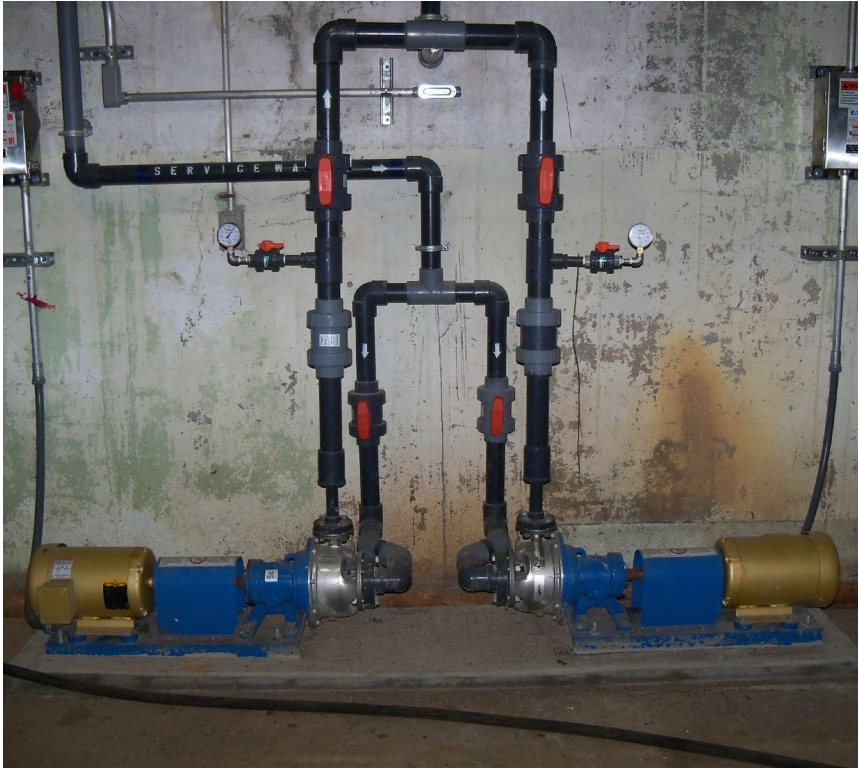
Wash Water Pumps
