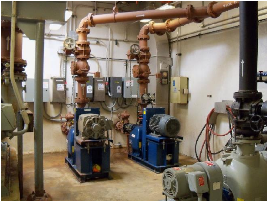
Waste Activated Sludge Pumps Gorman Rupp Self Priming
