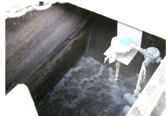
Overflow Influent Gate
