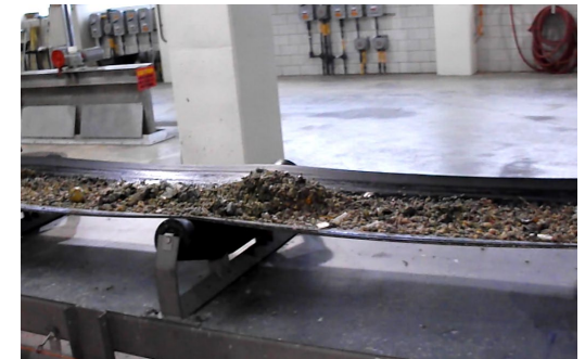
Screenings on Belt Conveyor
