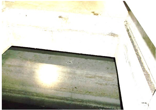
Freeboard before Test
