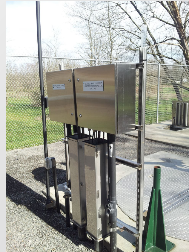
Terminal Box Installation Example
