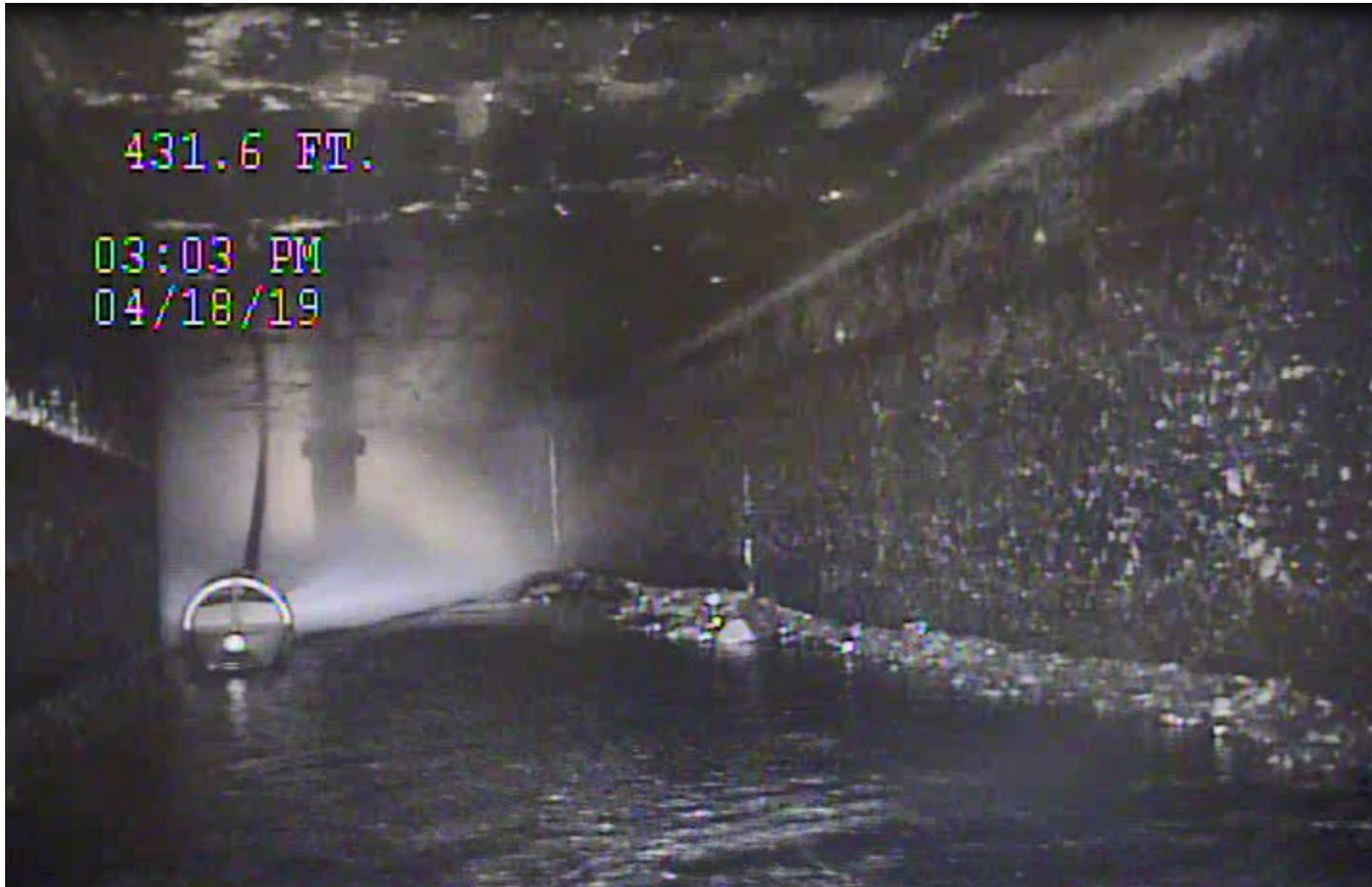
East Conduit Cleaning
