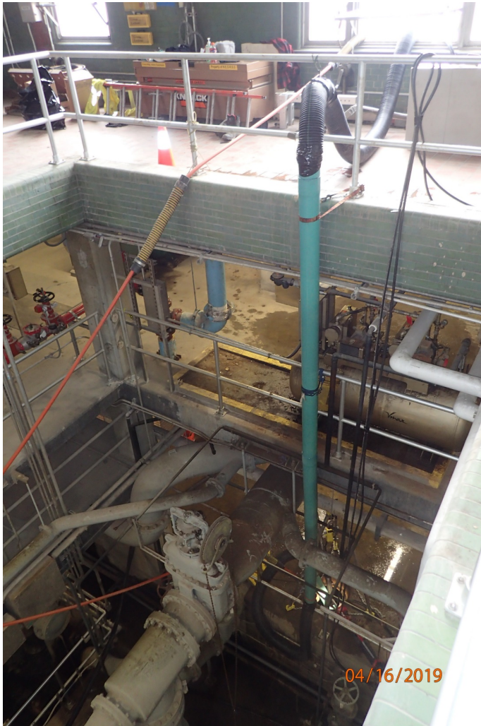
Vac Truck Suction Piping
