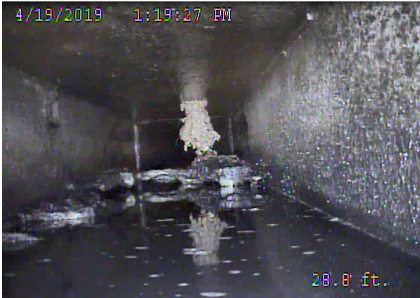
West Conduit Cleaning
