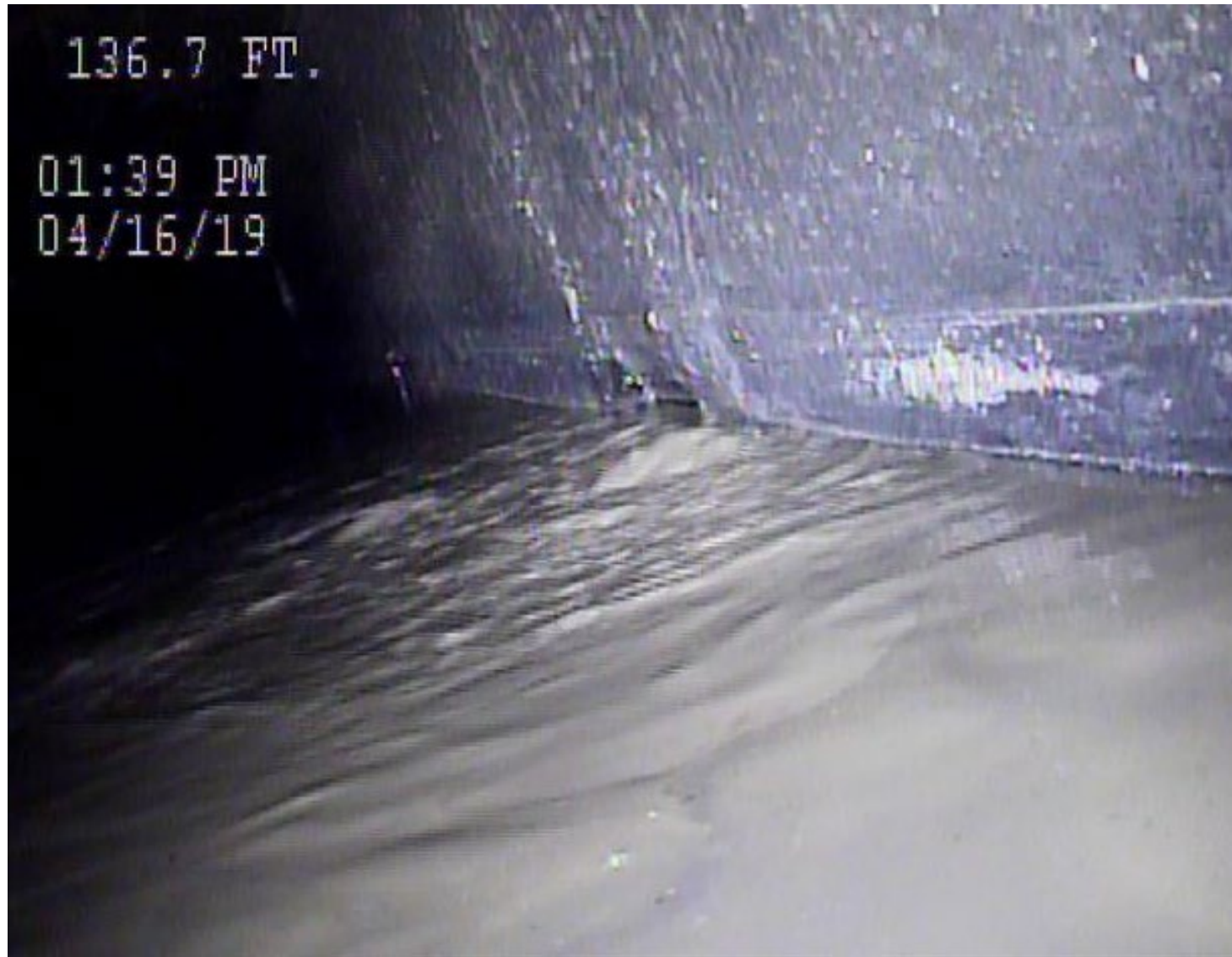
West Conduit South Wall Location A Leak
