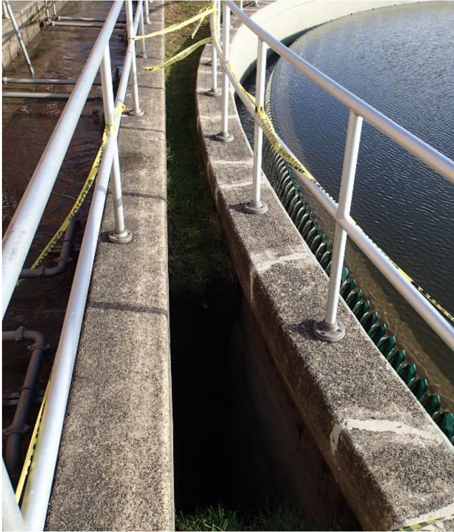
January 2017: Sinkhole Observed
