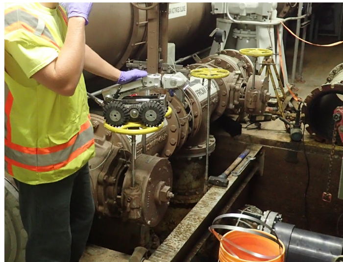
16" RAS piping in the Gallery was removed for remote camera access
