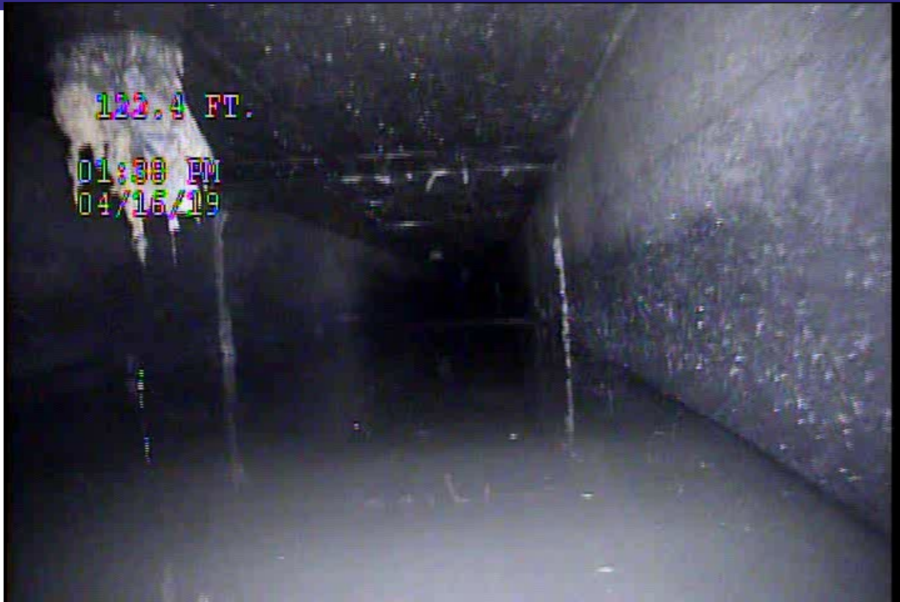
West Conduit South Wall Location A Leak Video
