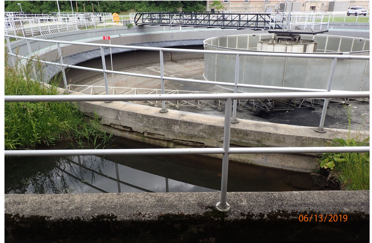
Pipe breaks were found directly below the sinkhole at FST 11
