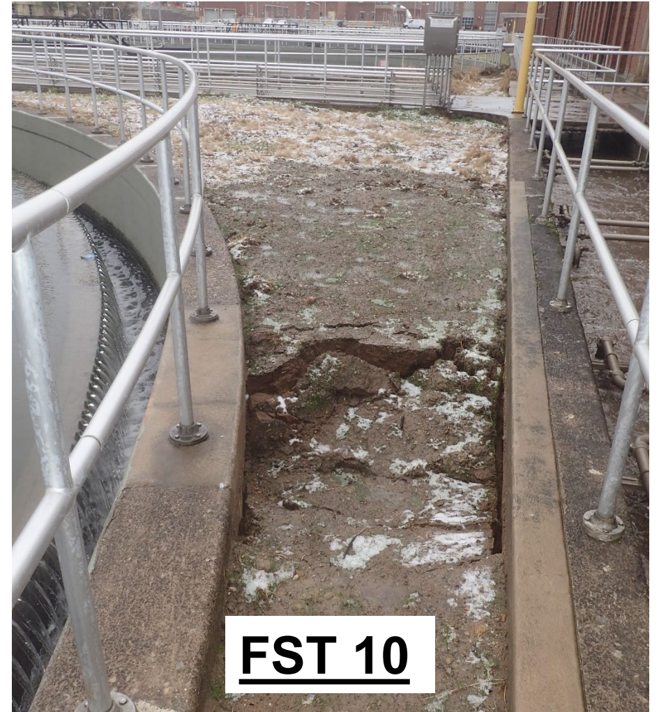
February 2018, Sinkhole Reappears (23 months after backfilling repair with sand)
