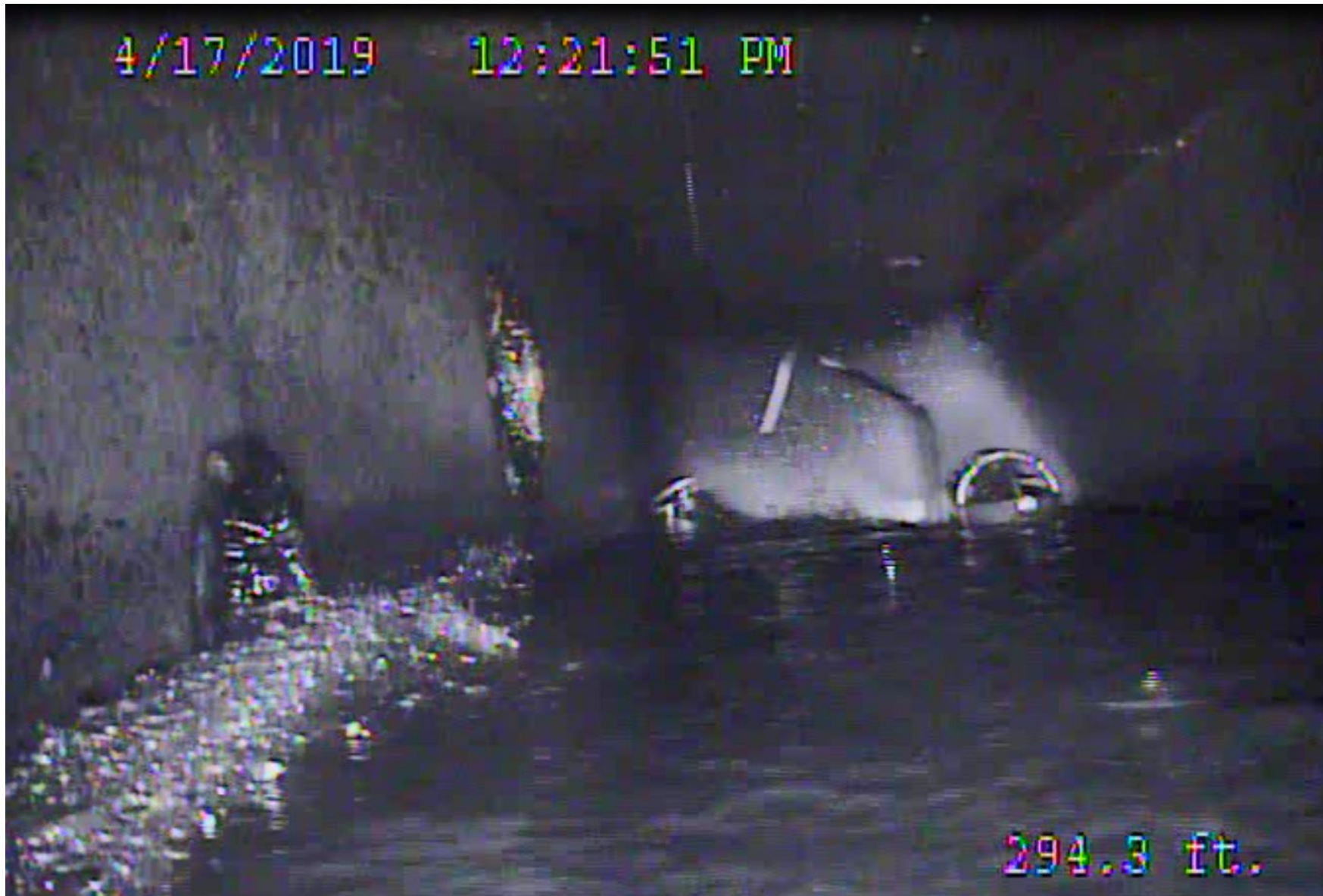
East Conduit Cleaning
