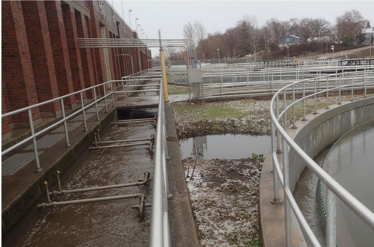
FST 11: Sinkhole appears in 2018
