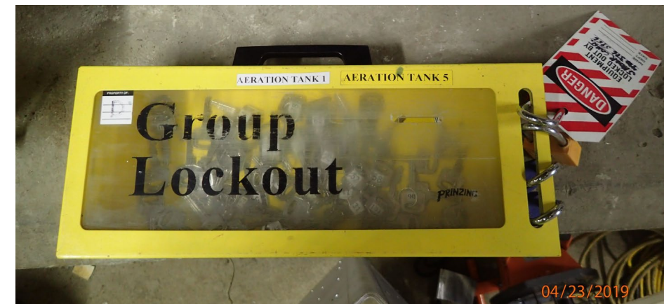
62 Valves Required Lock-Out
