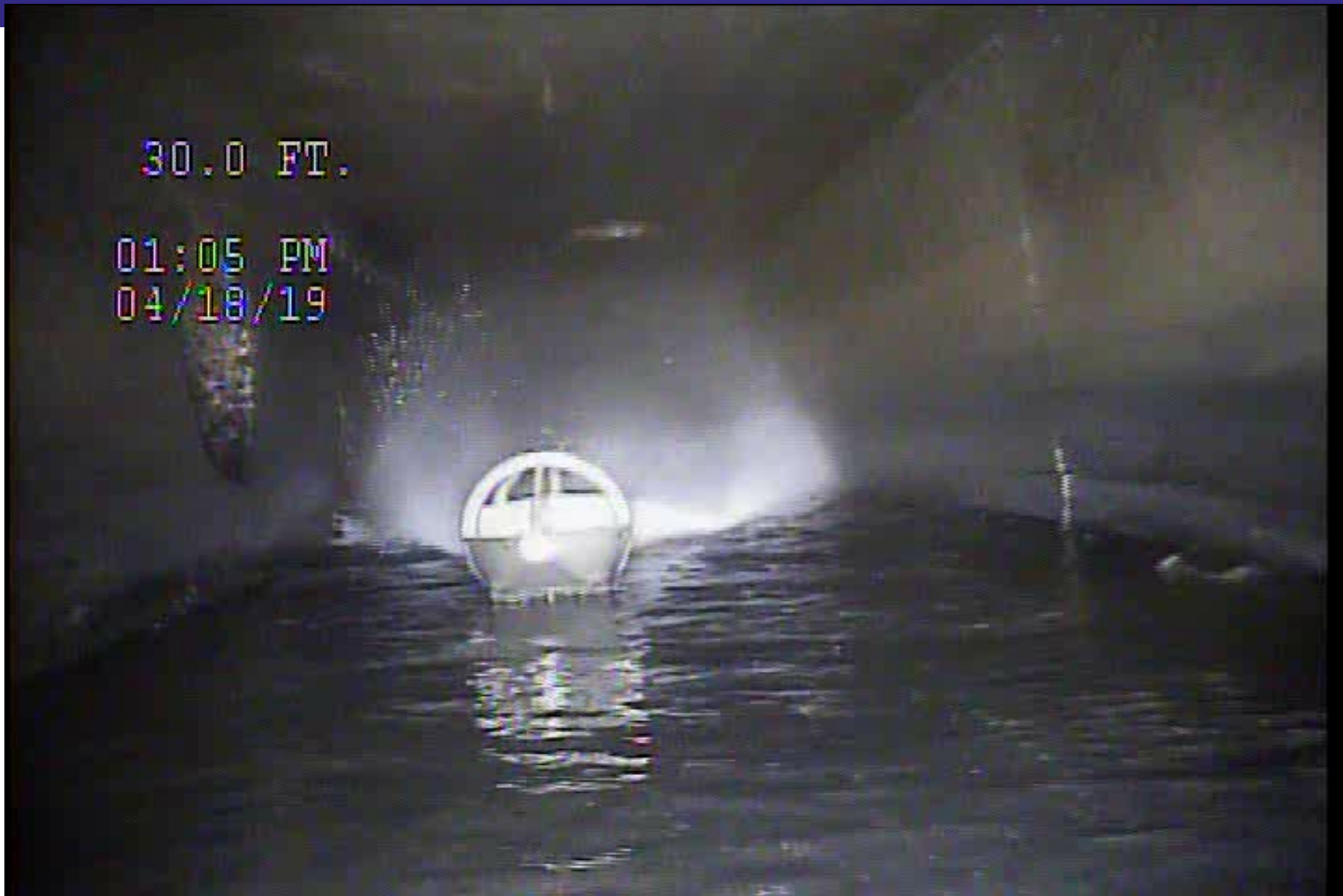
East Conduit Location C Leak Video
