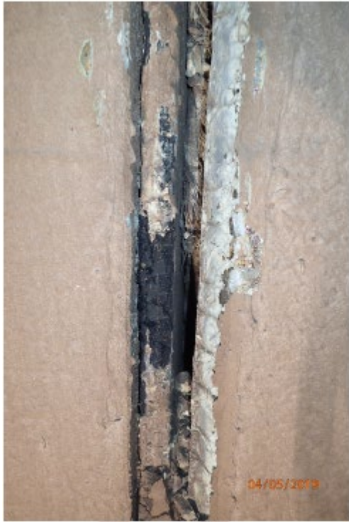
Expansion Joints Inside Discharge Conduit
