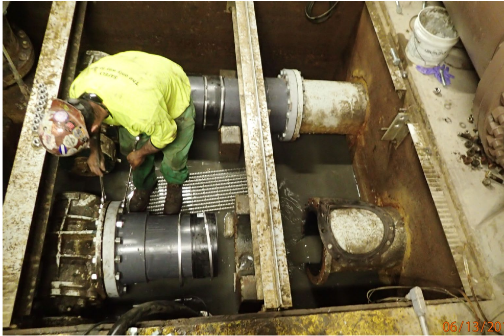
16" RAS piping in the Gallery was removed for remote camera access
