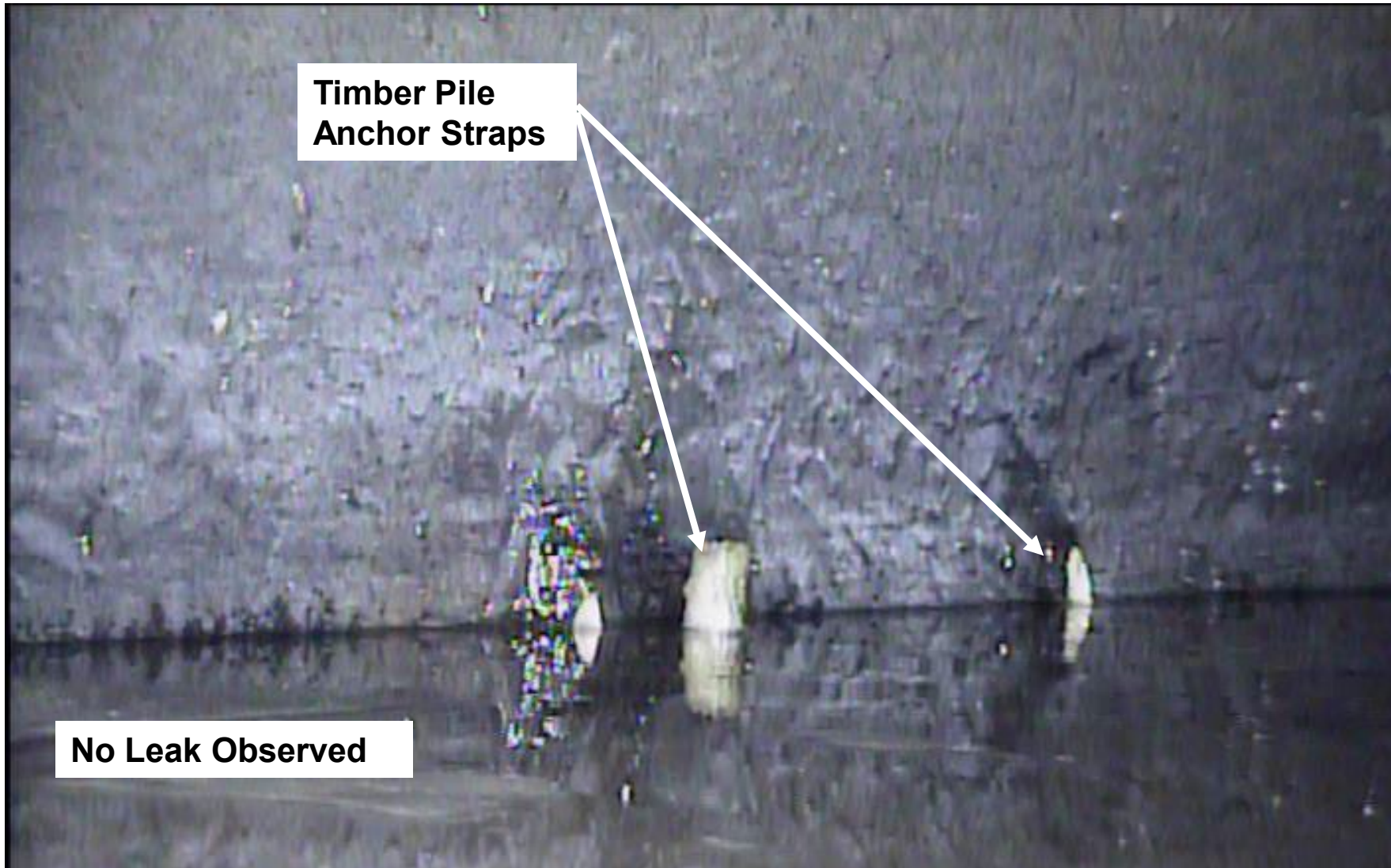
West Conduit North Wall Opposite Location A Leak
