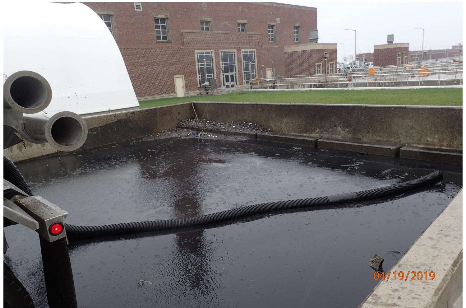
Grit Pad used for disposal of Vac Truck Contents
