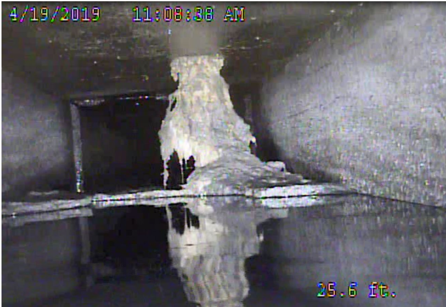
West Conduit Cleaning
