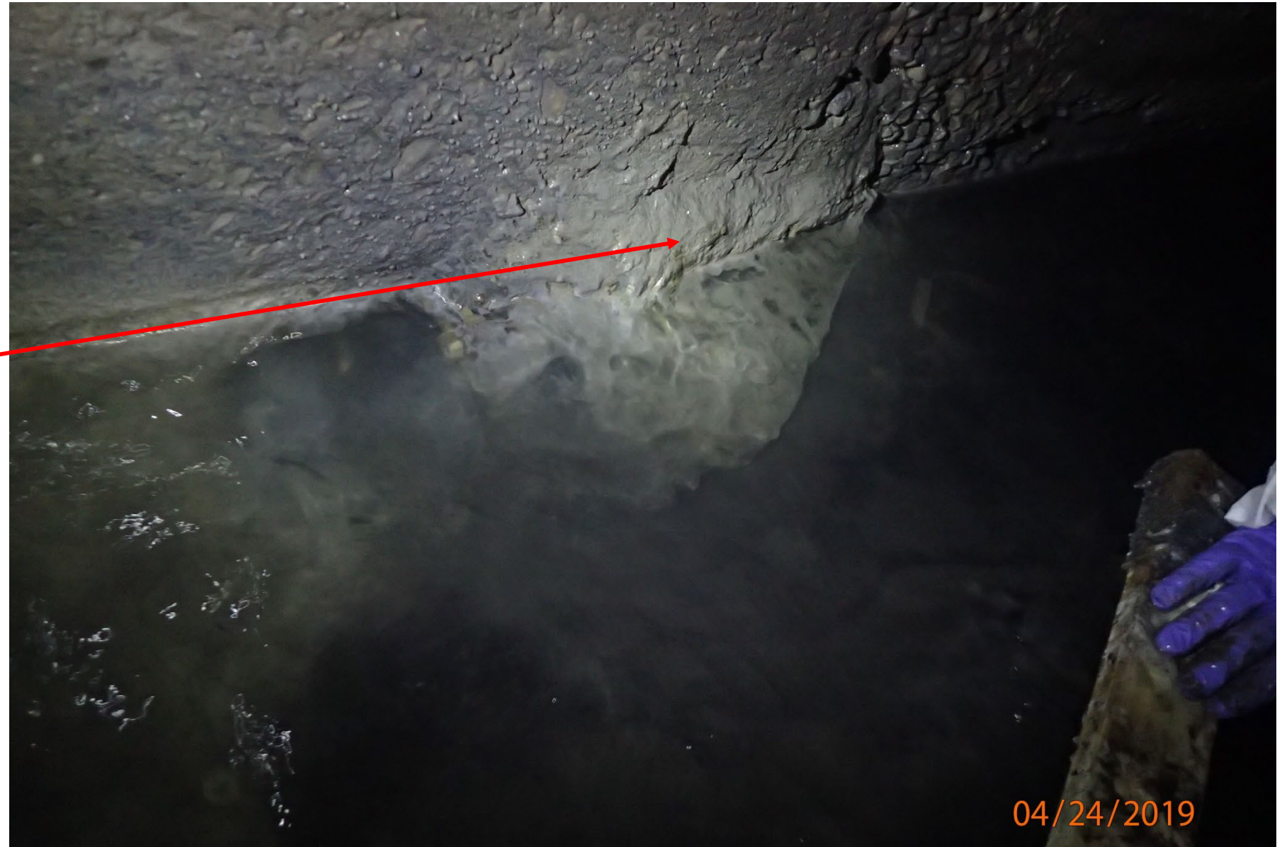
East Conduit Location C Repair
