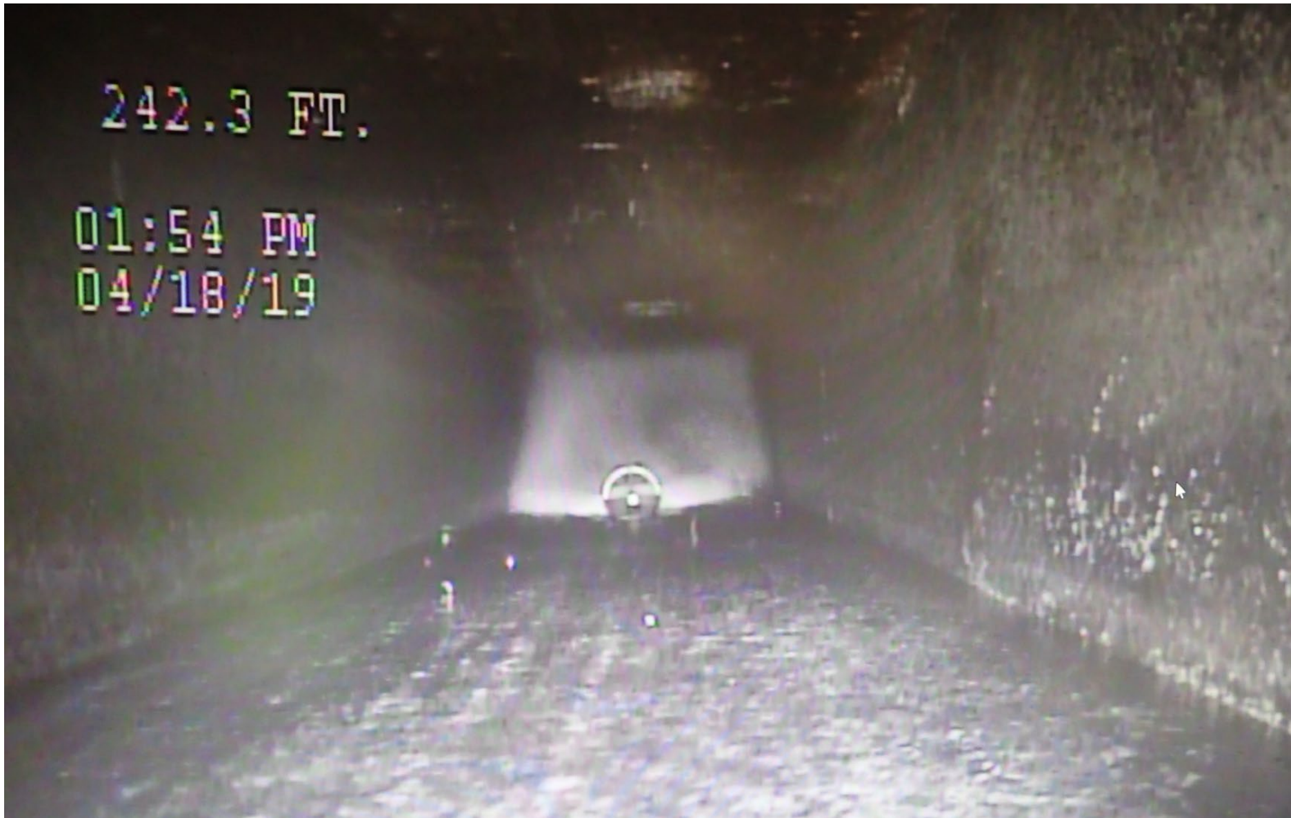
West Conduit Cleaning
