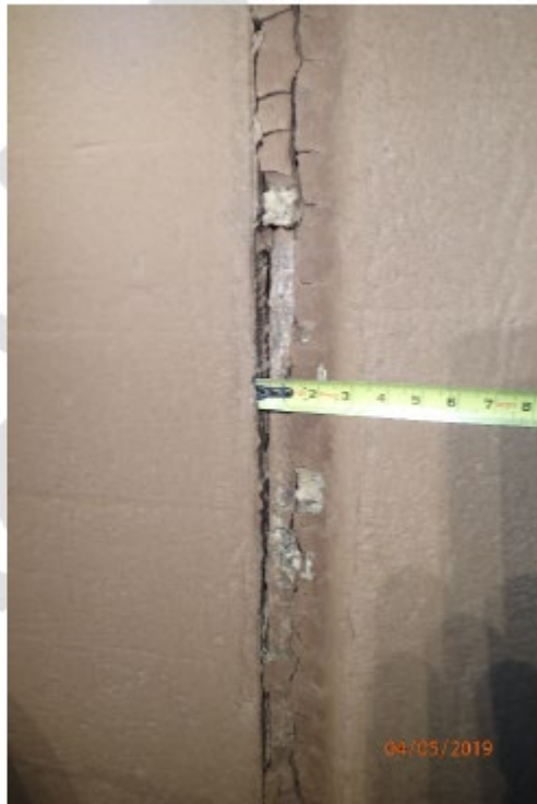
Expansion Joints Inside Discharge Conduit
