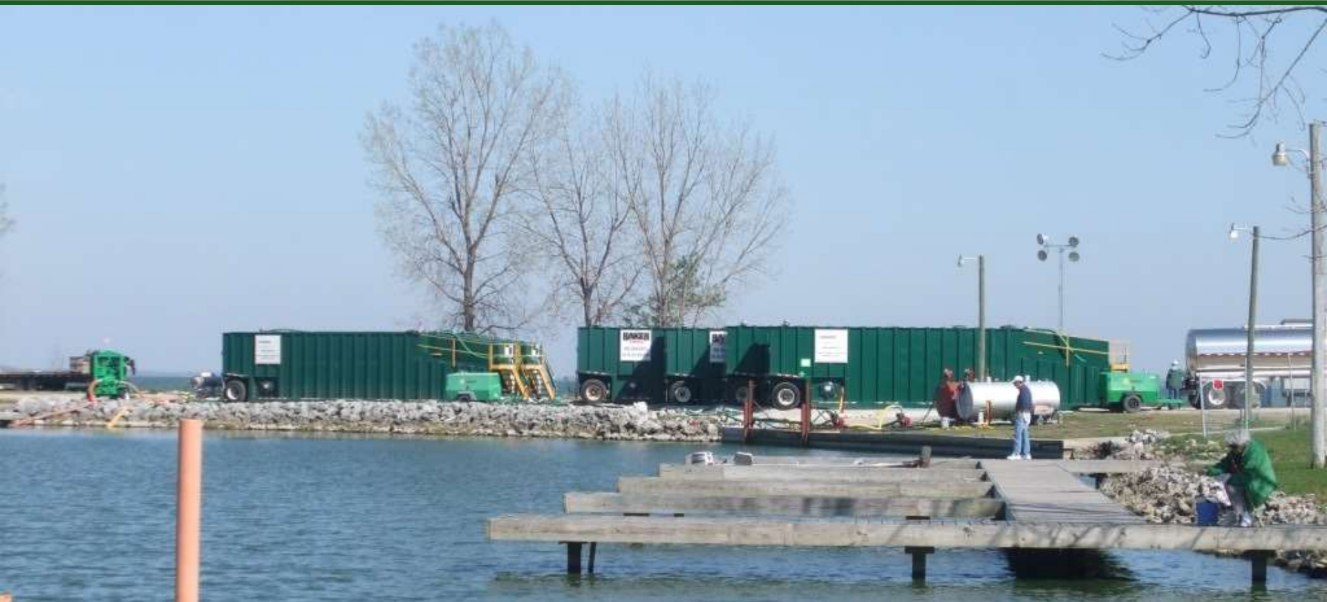
West End Staging Site
