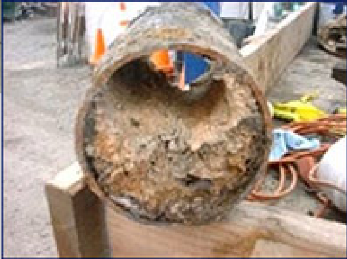
Hardened fats, oils and grease clogged a larger sewer pipe.
