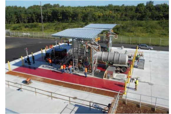
Truck Loading Station
