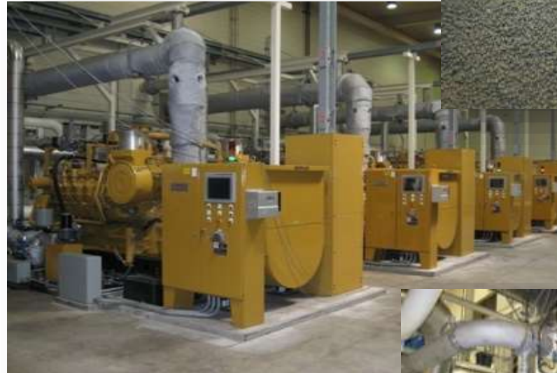
Four 750 kW Engine-Driven Generators, Rotary Drum Dryer
