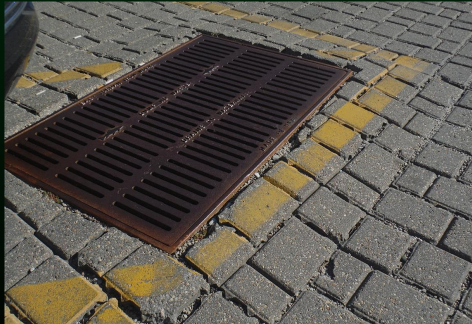
Frost Heave of Pavers
