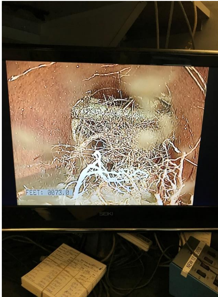
Cross bore with roots
