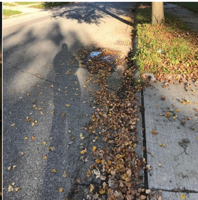
Pavement depression at collapse site
