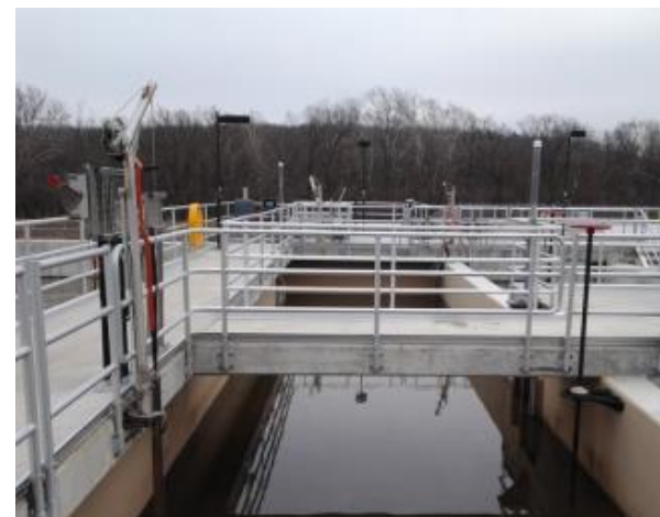
Off-line Fermenter with 5-stage Bardenpho 5.3-mgd Cedar Creek WWTP (Olathe, Kansas)
