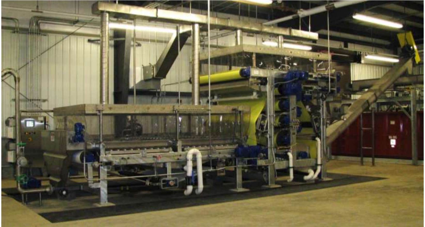
Odor Control Hoods for Belt Press
