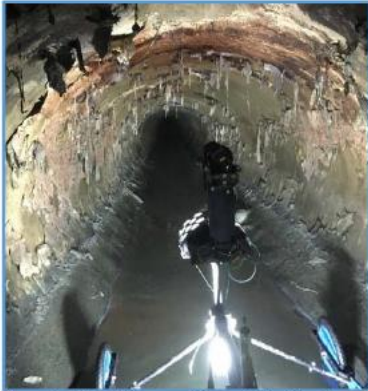
Photo 2.13 – “Swamp Buggy” inside the pipe
