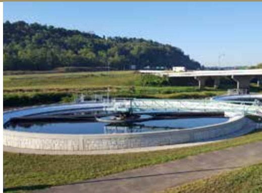
Wastewater Treatment Plant | Athens, OH
