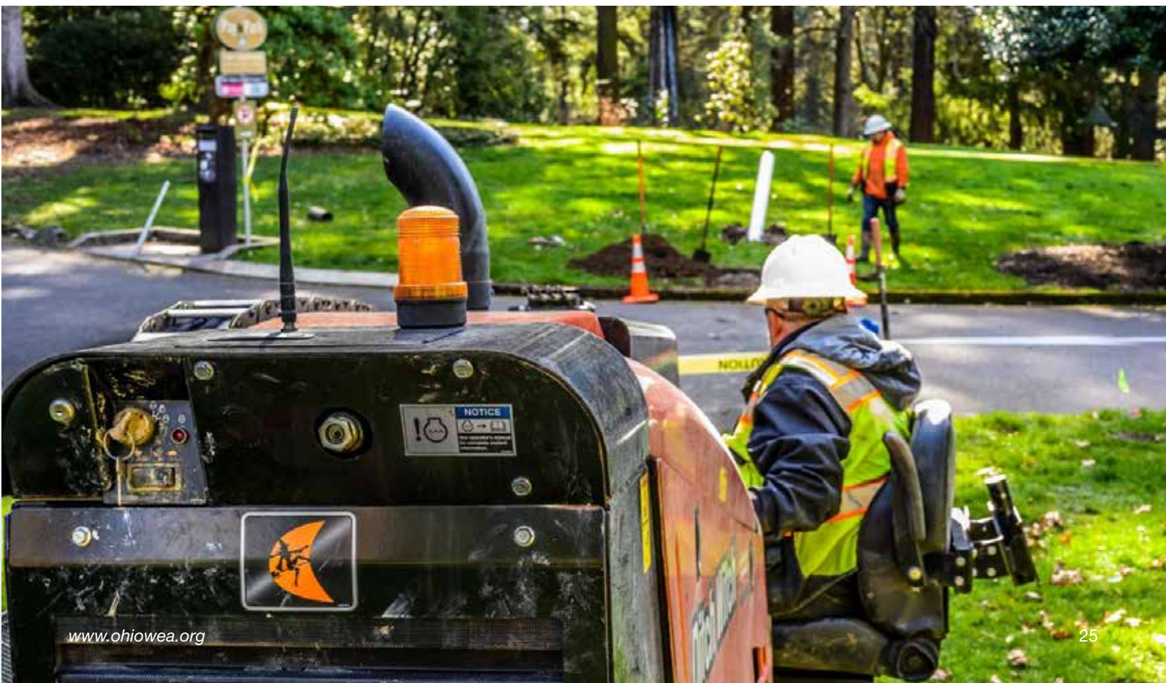
Figure 1 - Directional drilling under a road, showing equipment in foreground and pipe on opposite side of the road, which has been directionally drilled, in background.
