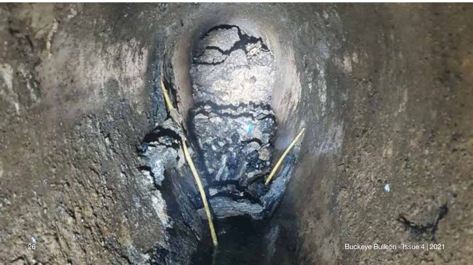
Figure 2 - Fatberg causing blockage of sewer.
