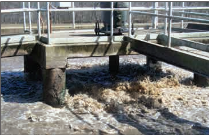
Mechanical aerator platform prior to rehabilitation
