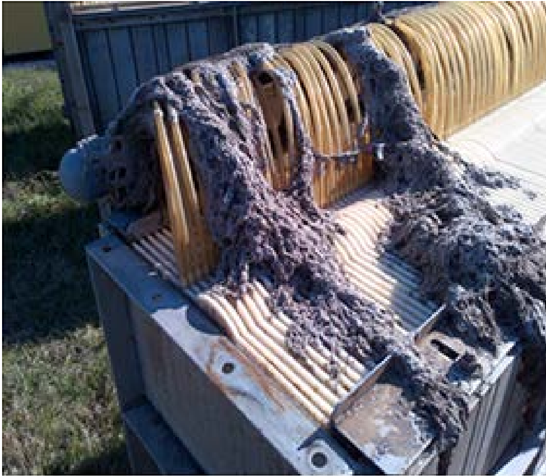
Material from a clogged MBR system
