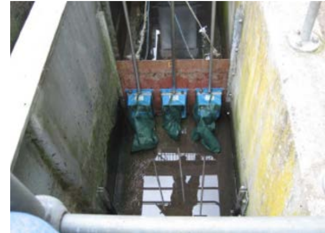
Debris that passes screen is collected in Copa Sacs
