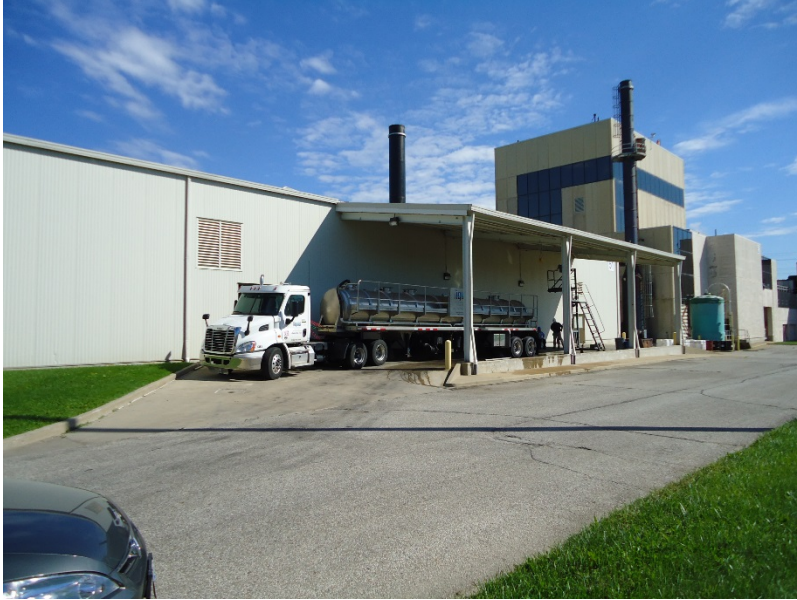
Existing DAFT and Skimmings Facility
