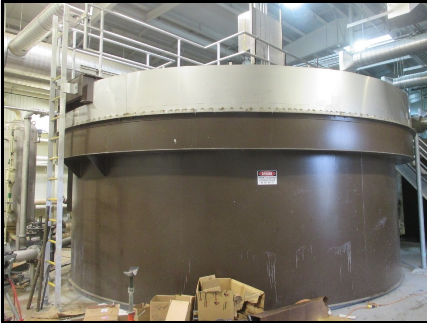
DAF Tank contents transferred to CSKIM Tanks
