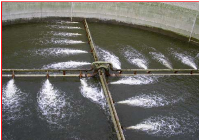
JET MIXING IN EQUALIZATION TANKS
