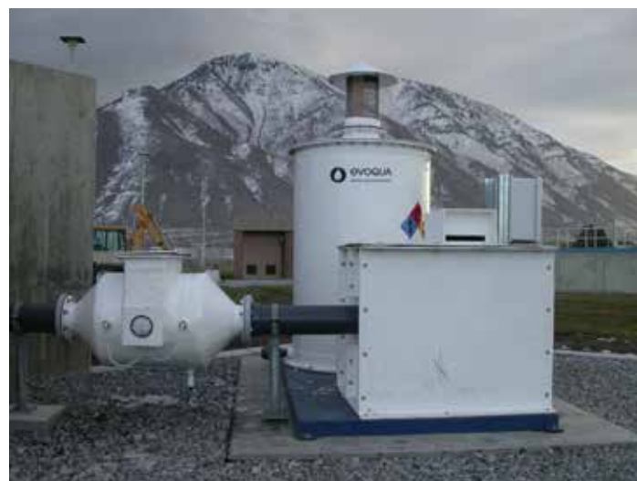
Carbon adsorption is the simplest of the vapor-phase technologies, with no required chemical storage and feed system, and no biological process to maintain. (RJMC Modular Carbon Adsorber)
