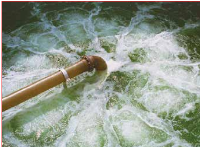
MIXING AND AERATION IN pH CONTROL TANK
