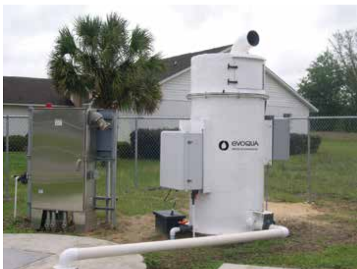
With a manufactured biological odor control system, media instability is reduced and control issues are limited. (ZABOCS® Biological Odor Control System)
