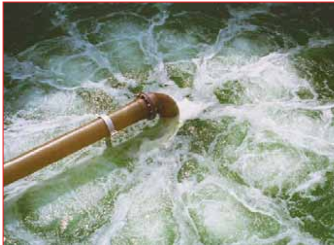
MIXING AND AERATION IN pH CONTROL TANK
