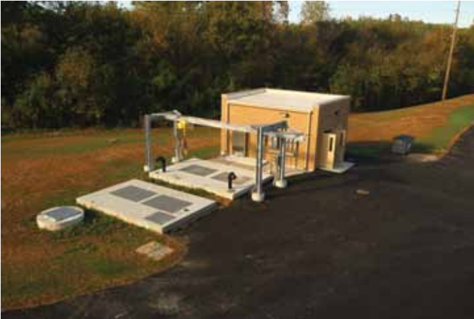
New Influent Screen Building and Submersible Pump Station
