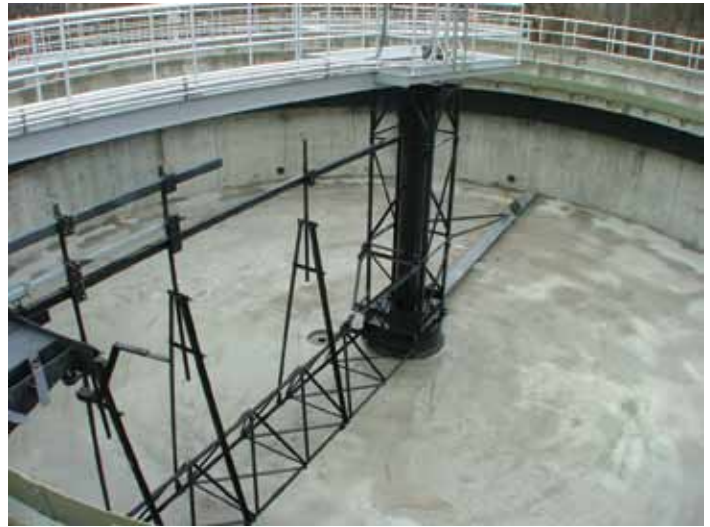
Final Clarifier Showing Suction Header
