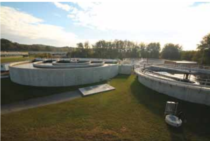
Oxidation Ditch and Final Clarifiers
