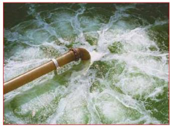
JET MIXING IN EQUALIZATION TANKS
