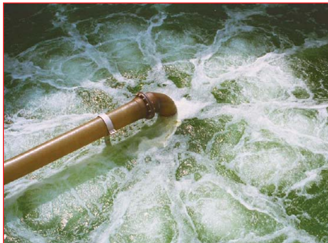
MIXING AND AERATION IN pH CONTROL TANK
