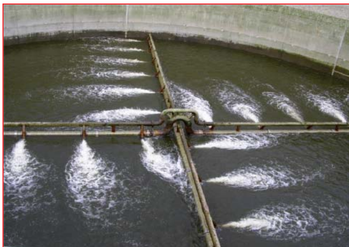
JET MIXING IN EQUALIZATION TANKS
