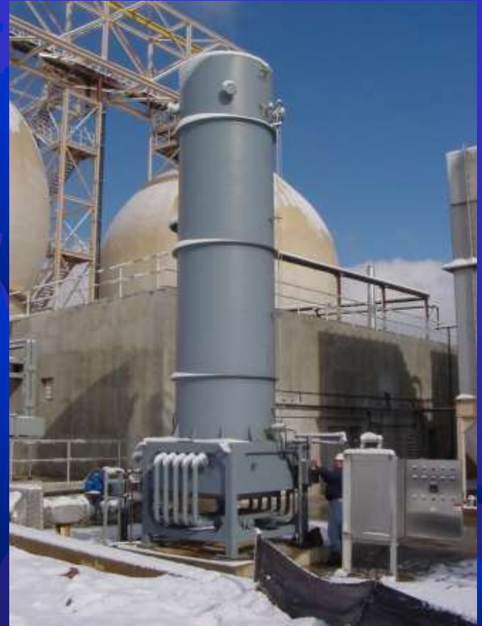
F. Wayne Hill Water Resources Center, Gwinnett County, GA
