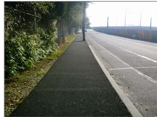
Philadelphia Zoo – Sidewalk on Zoological St. Porous Asphalt
