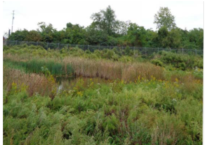
South 61 st St. Surface Detention Basin
