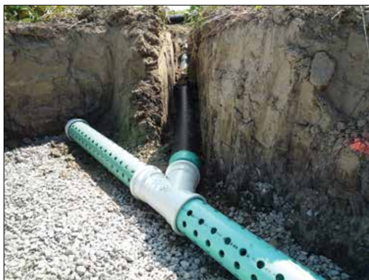
Installation of submerged vegetated bed outlet structure.
