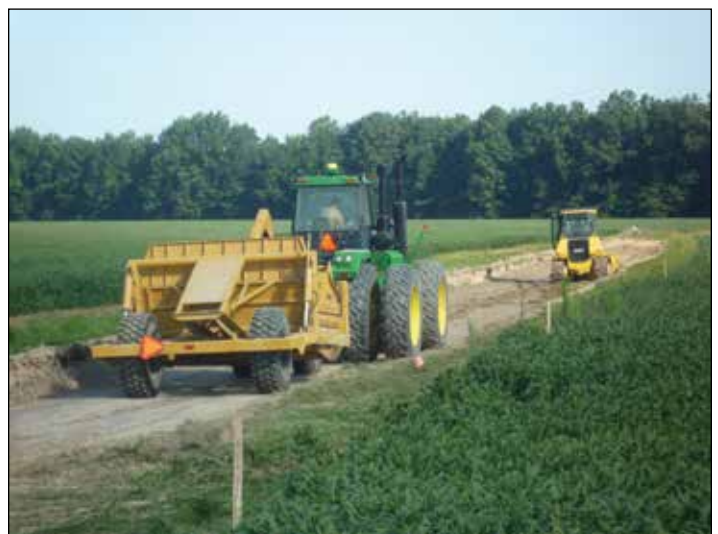
Excavation of AgBMP detention structure.
