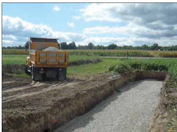
Placement of gravel in submerged vegetated bed.
