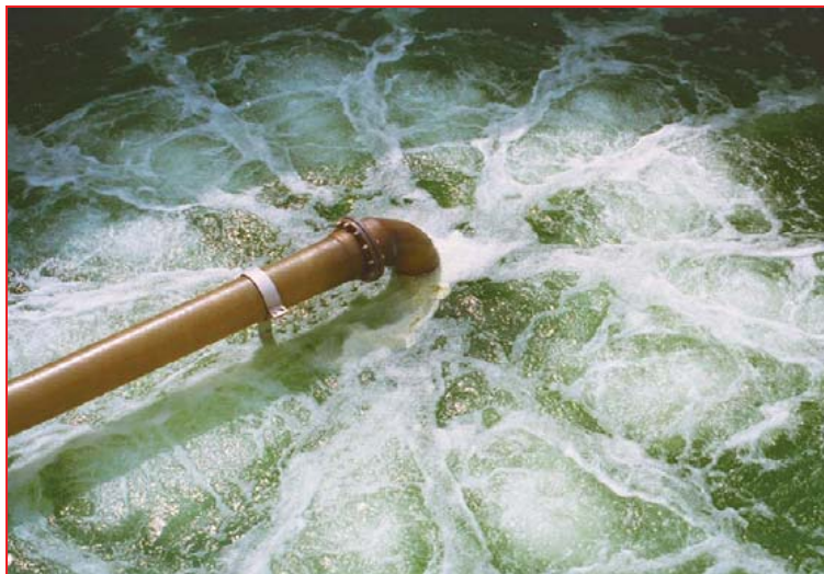
MIXING AND AERATION IN pH CONTROL TANK
