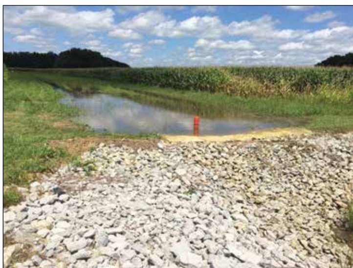
AgBMP detention structure after a summer storm.
