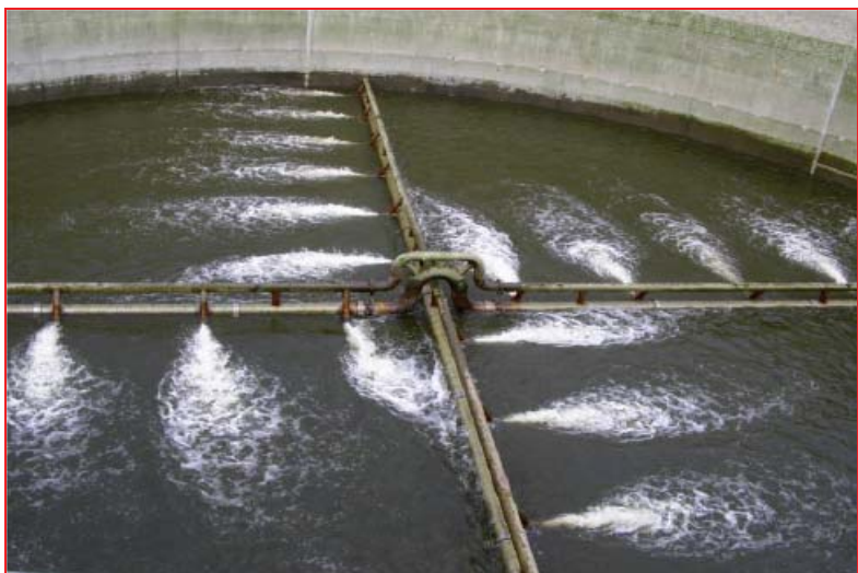
JET MIXING IN EQUALIZATION TANKS
