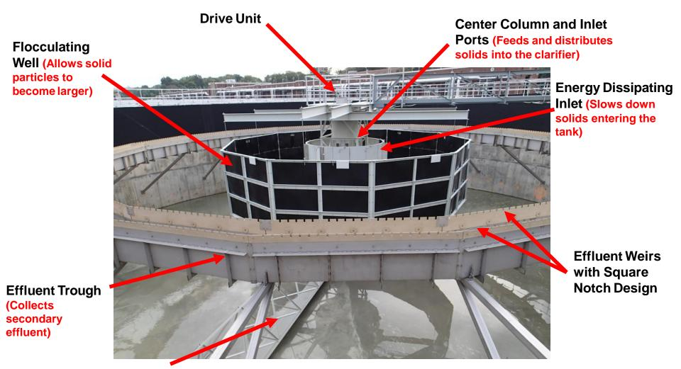
Sludge Collection Arm (Designed to rapidly remove settled solids)
