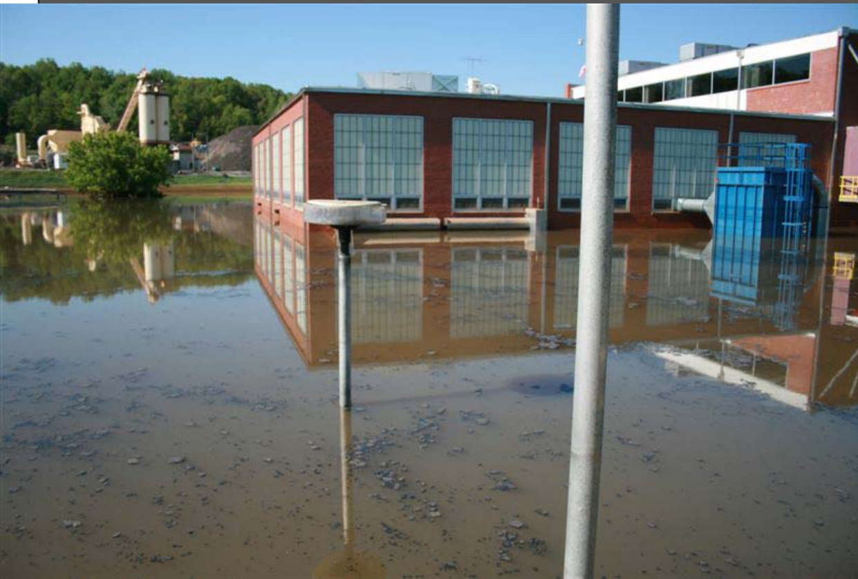
Clarksville WWTP: Solids Handling Facility May 6, 2010
