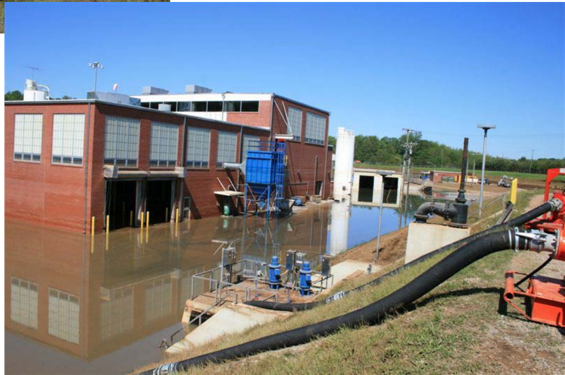
Clarksville WWTP: Solids Handling Facility May 9, 2010
