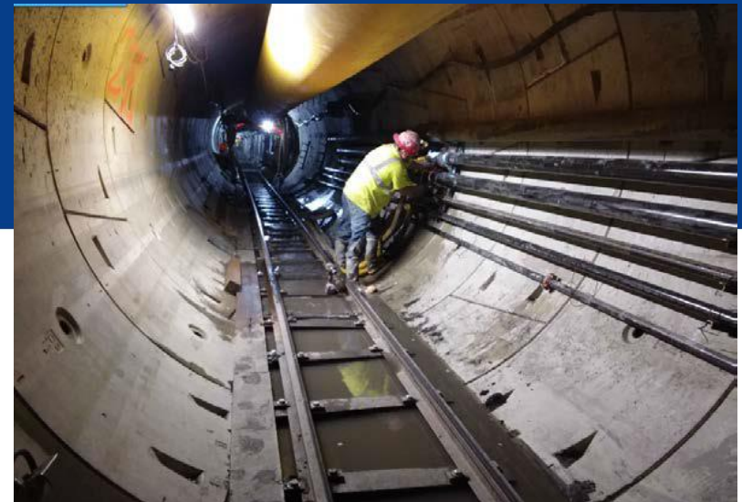
Utility Extension Work in Tunnel
